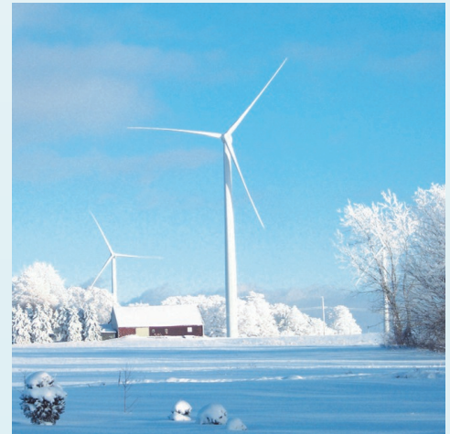
Photo Credit: Invenergy LLC, Wyoming County, NY
