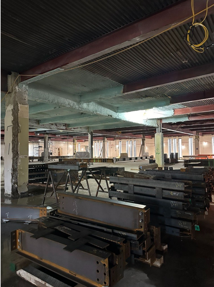
Rigging and installation of enabling Truss is ongoing. Bolting, rigging and welding to occur.
