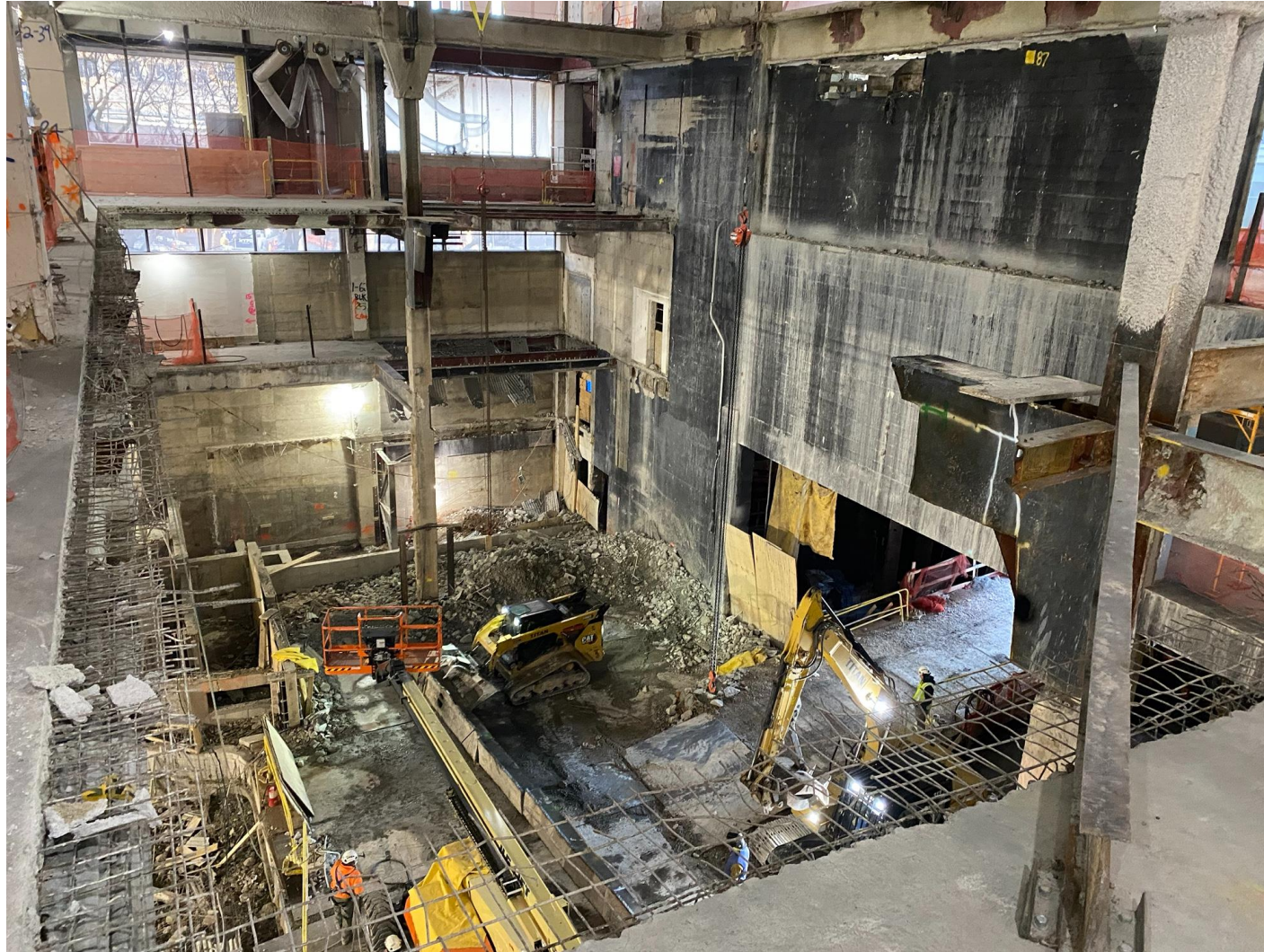
Large Venue girder truss has been completely demolished.
