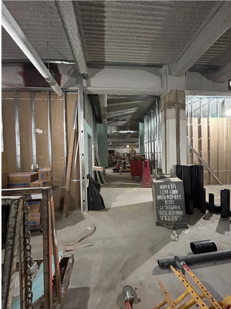
Framing, insulation and sheetrock installation on the 3 rd Floor in the Podium.
