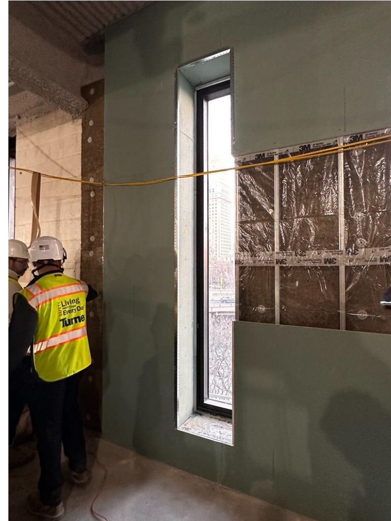
Framing, insulation and sheetrock installation on the 3 rd Floor in the Podium.
