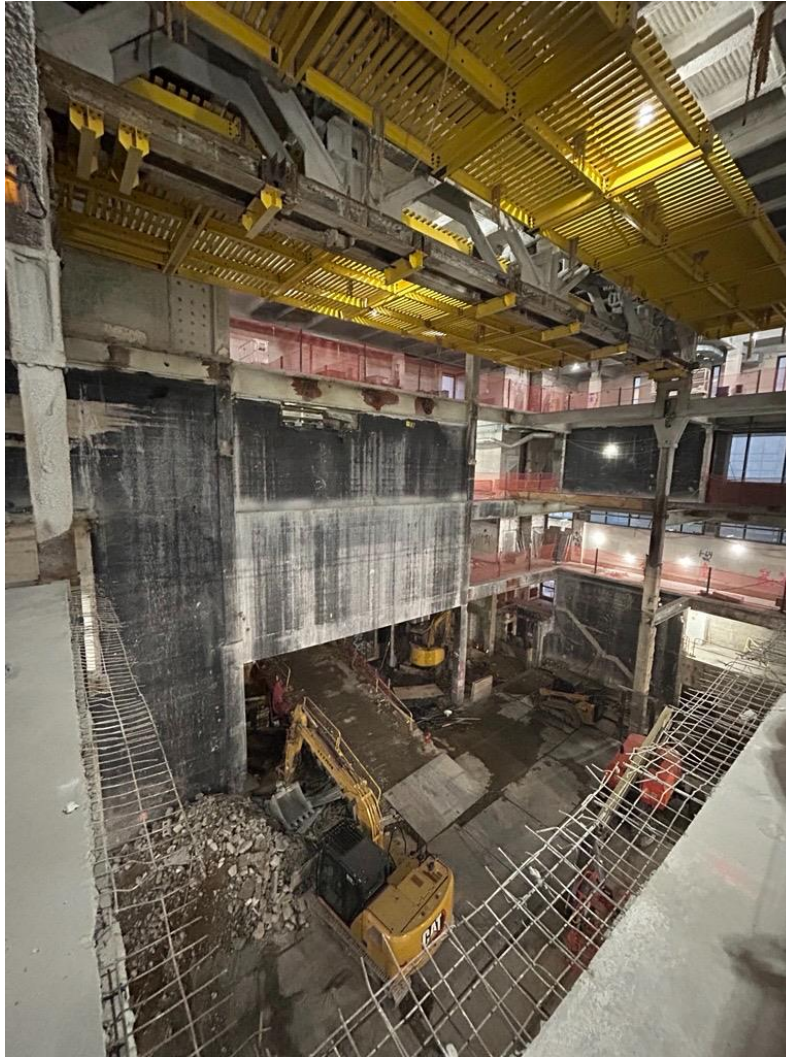
Large Venue structural demolition is substantially complete. Existing truss has been demolished.
