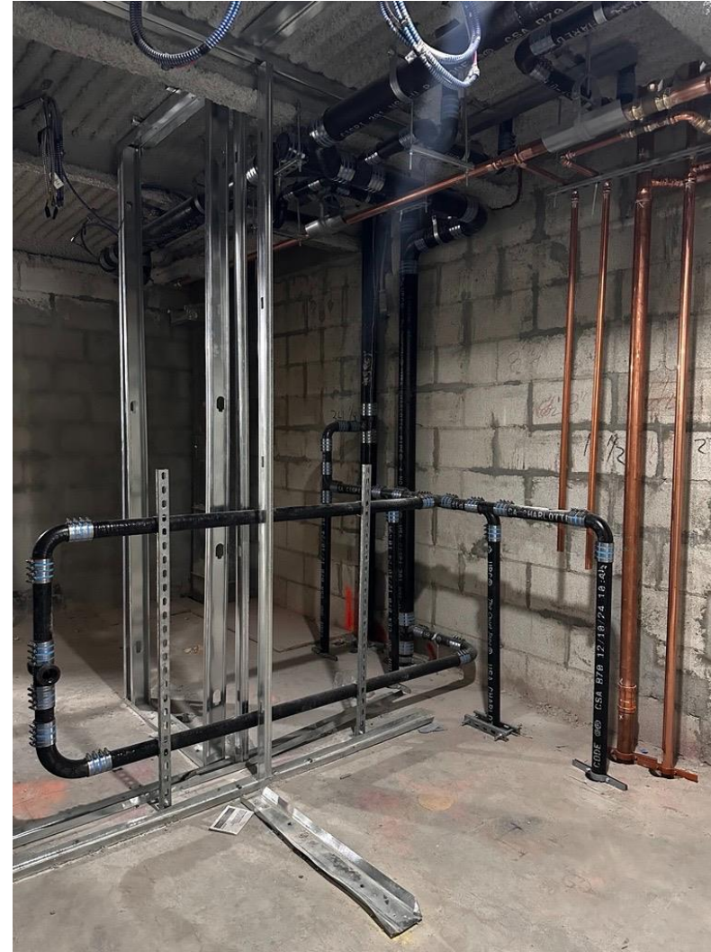
Maria's Tower bathroom framing and pipe installation.
