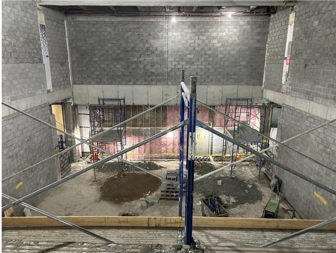
View of Small Venue from 1 st Floor.
