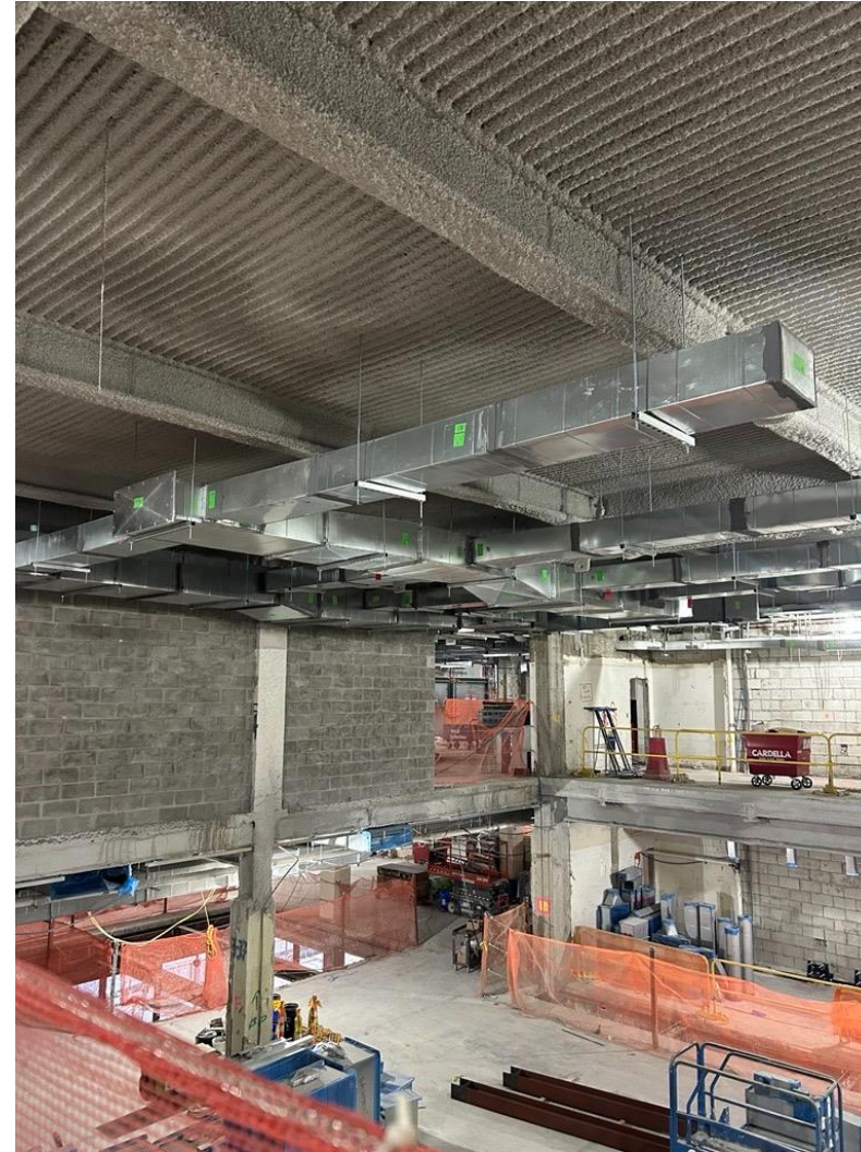
Installation of ductwork in the double-height dance rehearsal studio.
