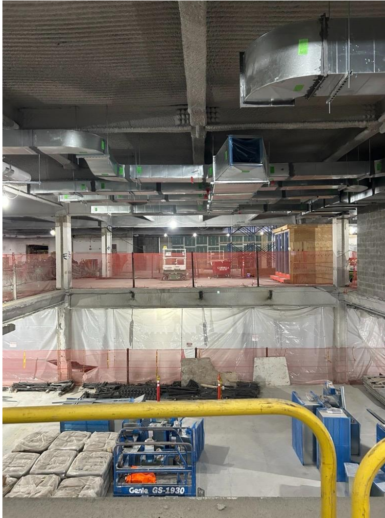
Installation of ductwork in the double-height dance rehearsal studio.
