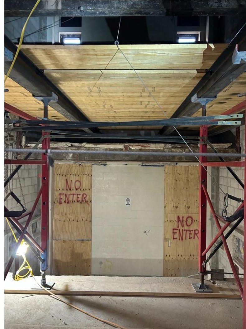
New freight elevator structural work has begun.
