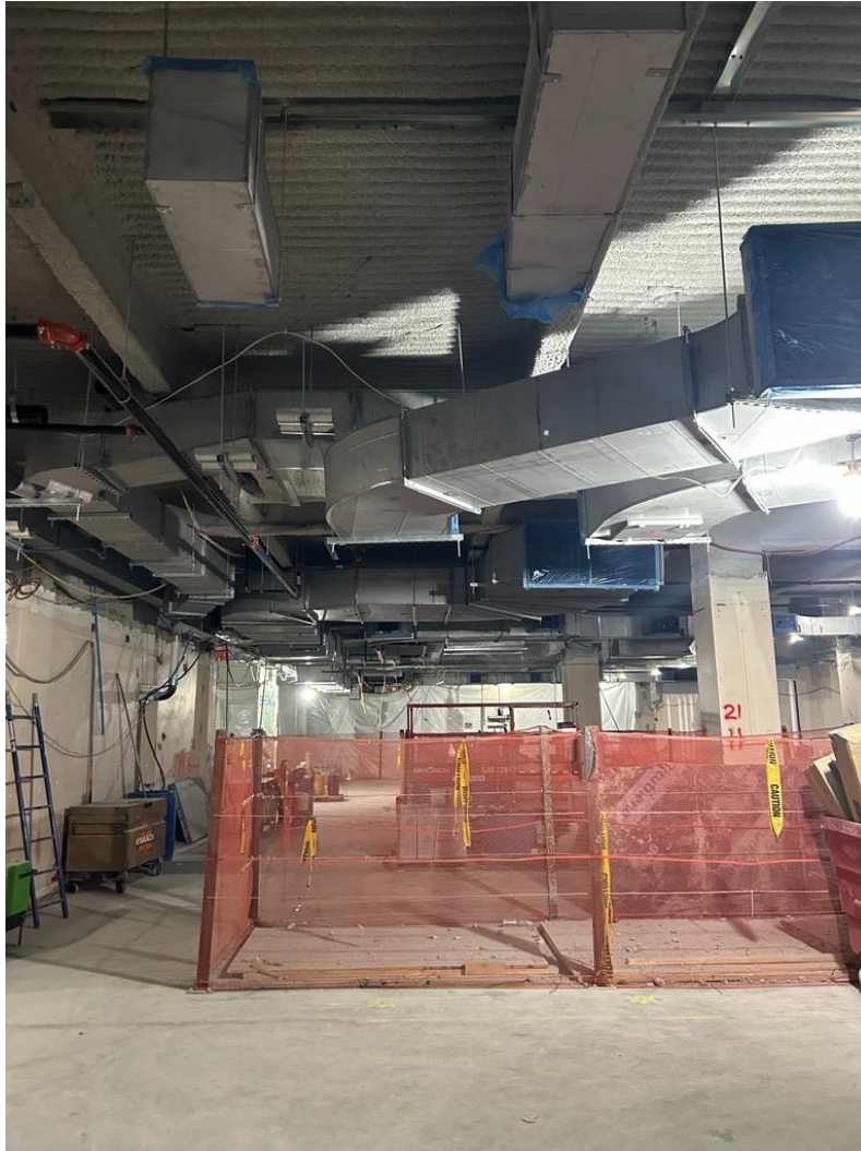
Overhead MEP installation on going on 1 st , 2 nd and 3 rd floors.
