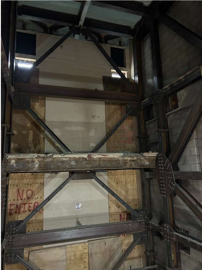
New freight elevator shaft steel installation.
