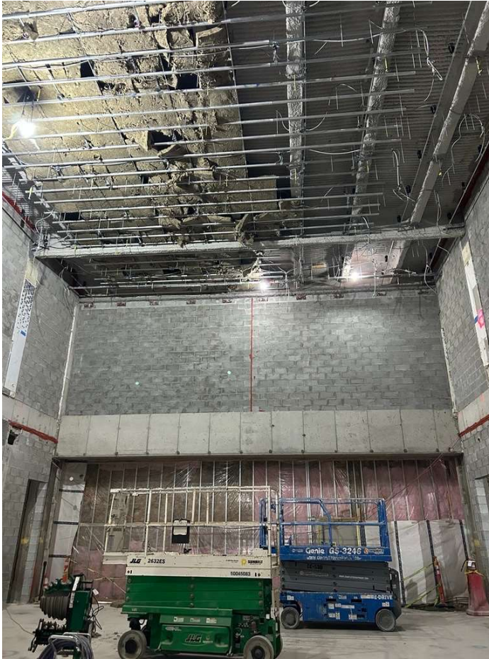
Small and Medium Venue conduit and hanger installation continues.
