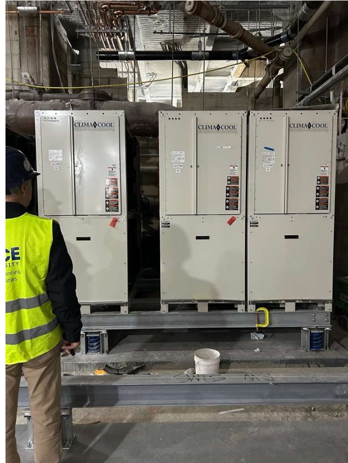
Cellar Water Source Heat Pump Installation
