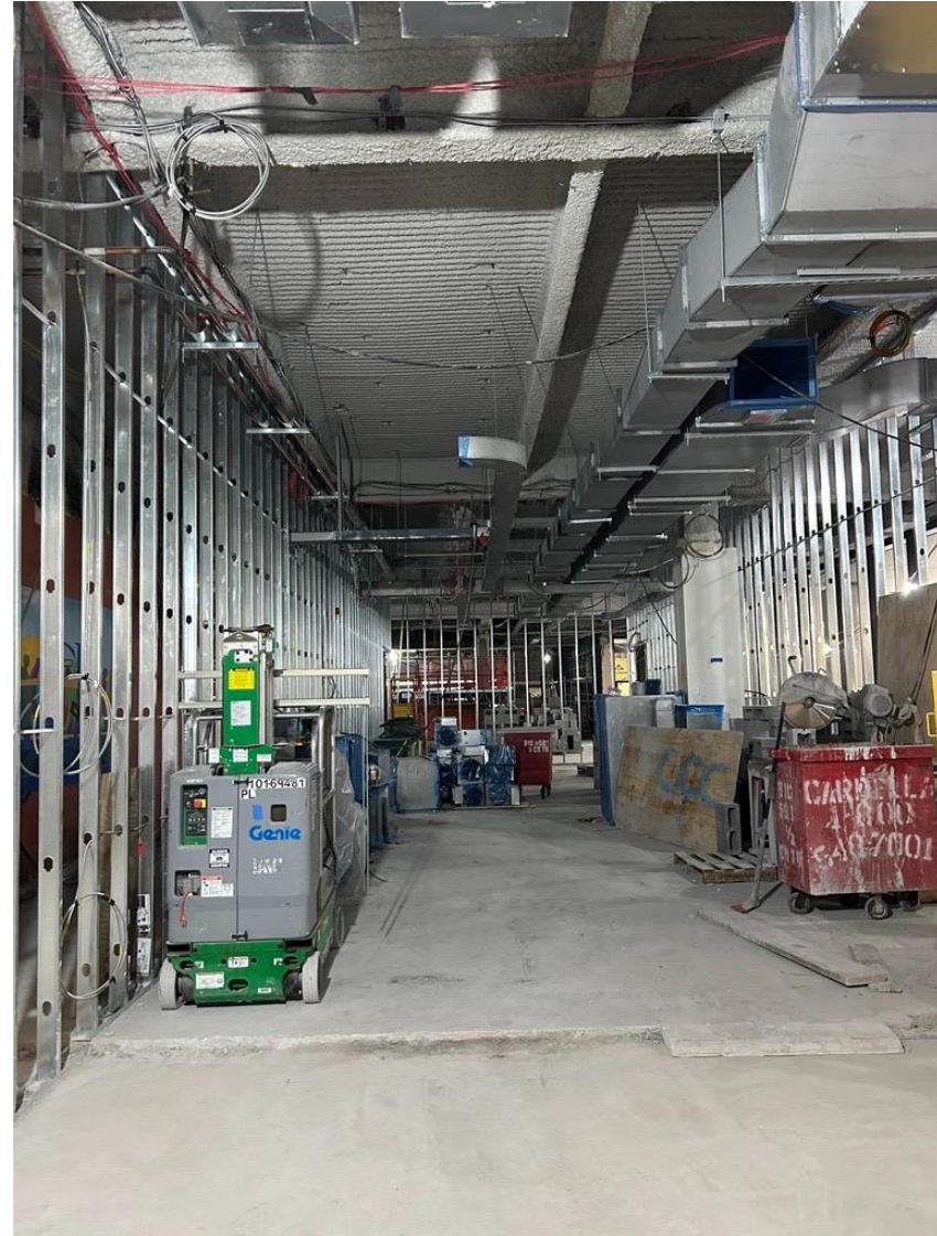
Framing and ductwork installation continues throughout the Podium floors.
