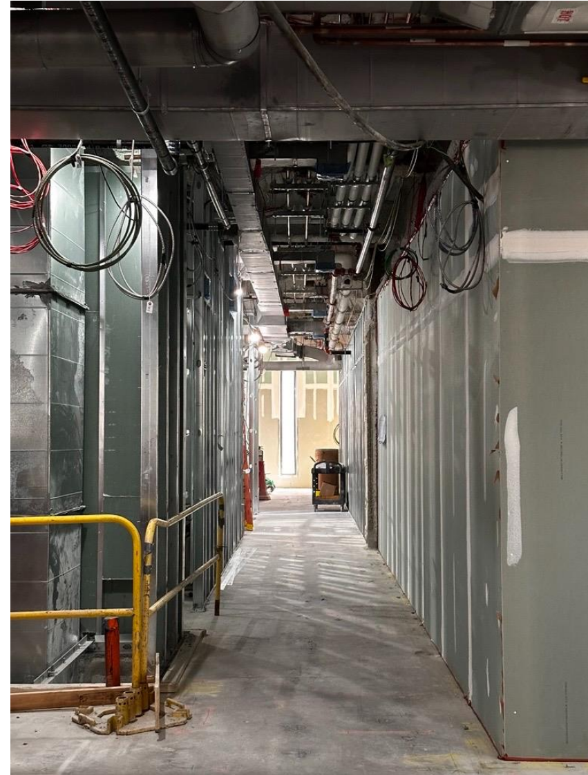
Gyp wall installation continues throughout the Podium floors.
