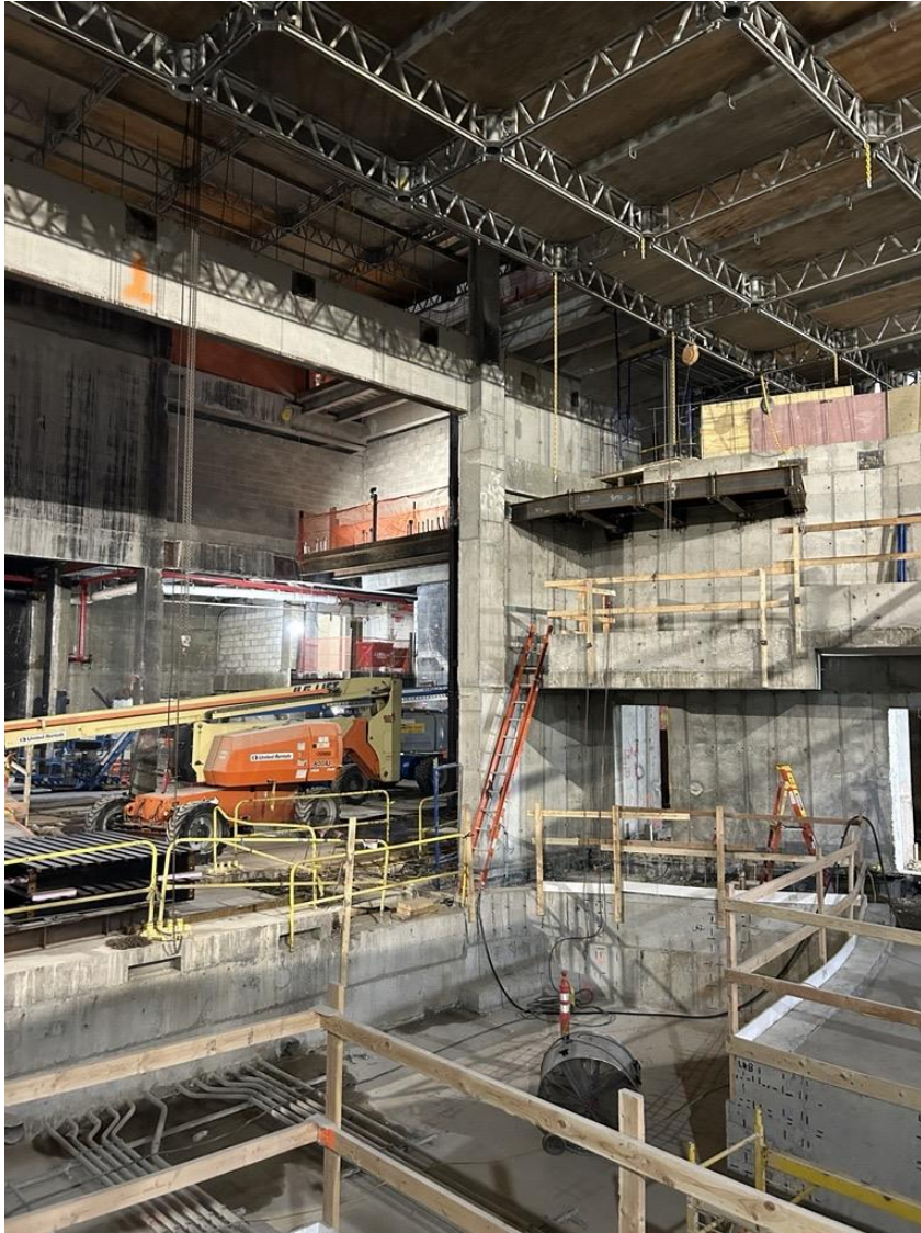
Ongoing concrete formwork and structural steel in the Schimmel Theatre.
