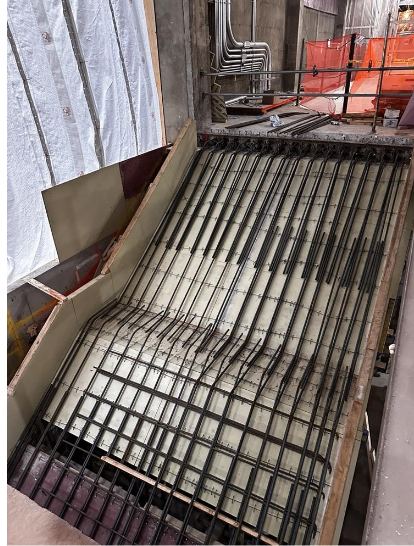
Rebar installation prior to concrete pour for the new feature stair.
