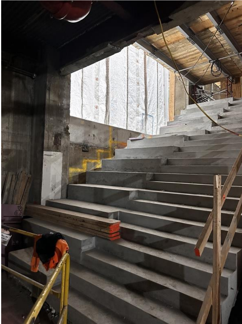
Installation of new feature stair “The Stoop” along the Spruce St façade is ongoing.
