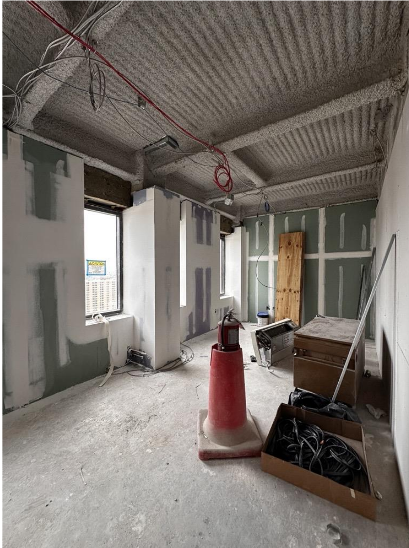
Installation of Maria's Tower dorm room gypsum walls
