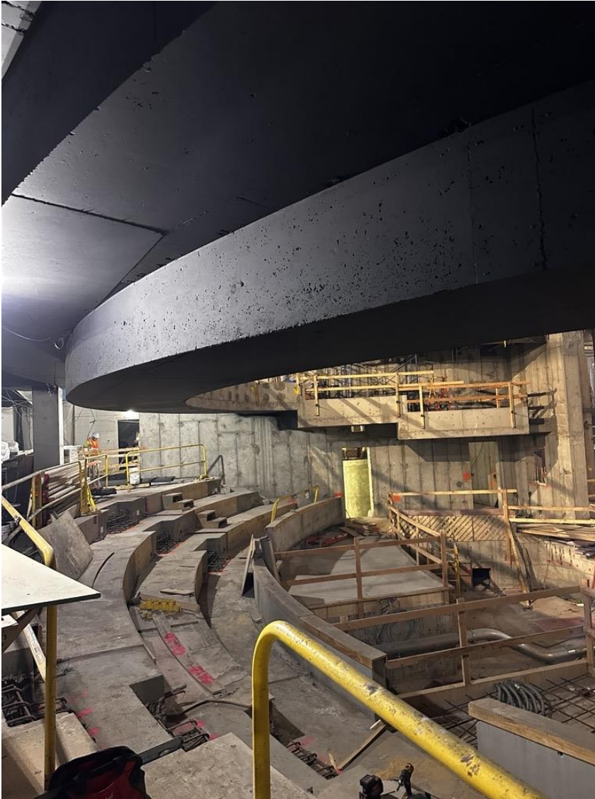
Concrete formwork and CMU installation continues in the Schimmel Theatre.
