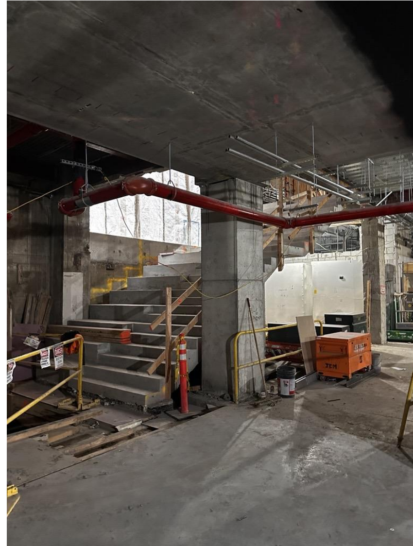
Installation of new feature stair “The Stoop” along the Spruce St façade is ongoing.
