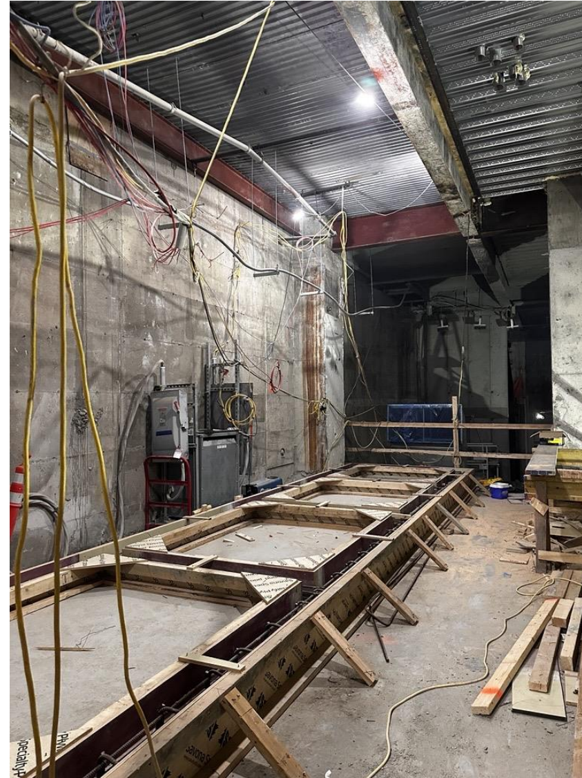
Installation of new concrete pads for new mechanical units.
