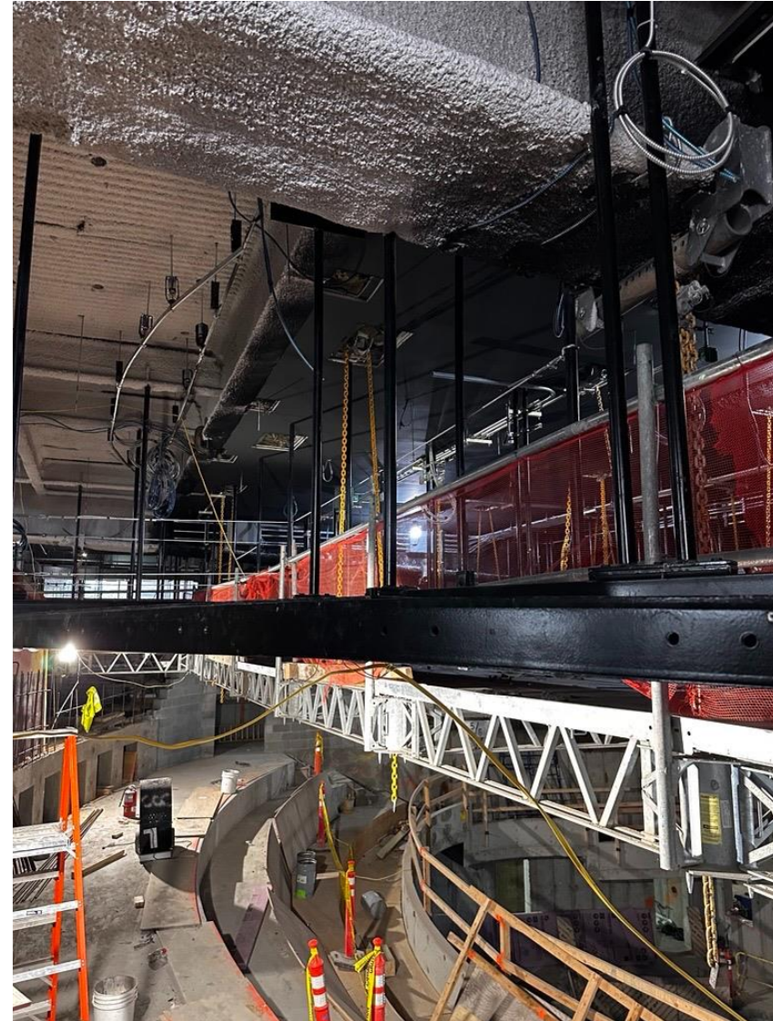
Installation of Schimmel Theatre Catwalk continues
