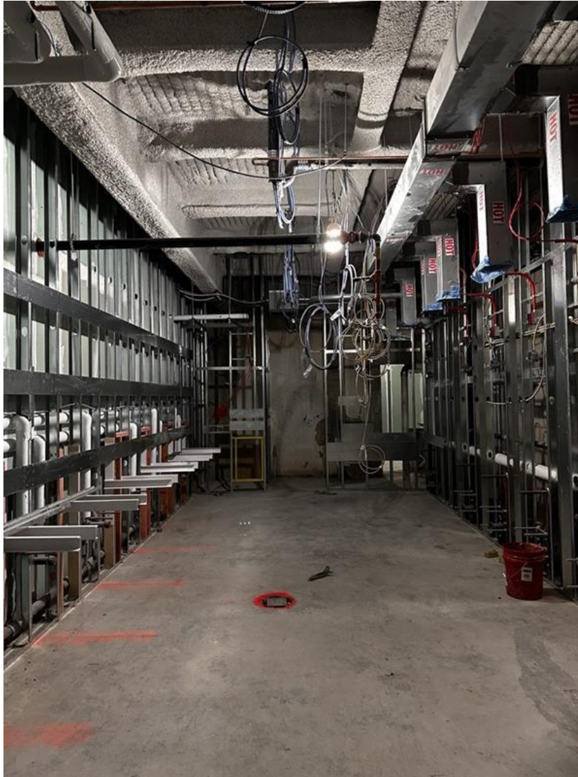
Installation of bathroom and dressing room gypsum walls and other interior trades continues
