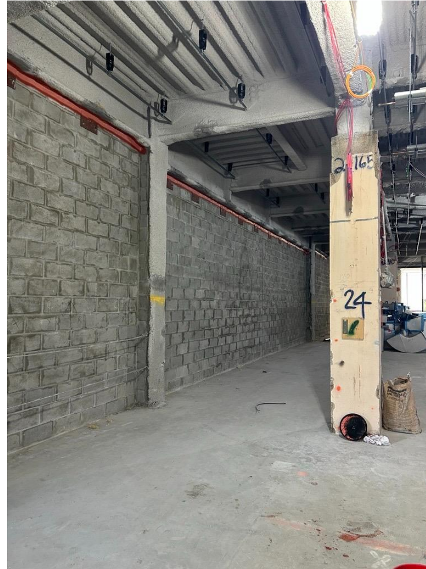
Firestopping on the 2 nd Floor
