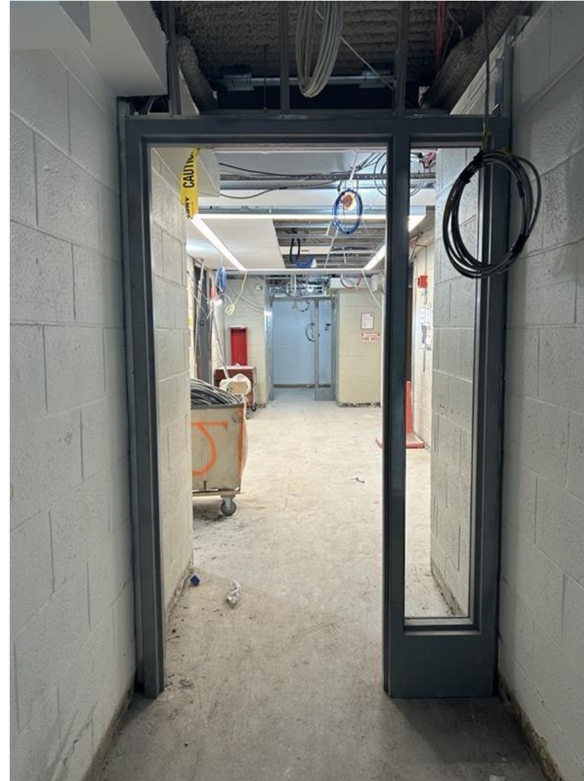
Maria's Tower elevator lobby door installation.
