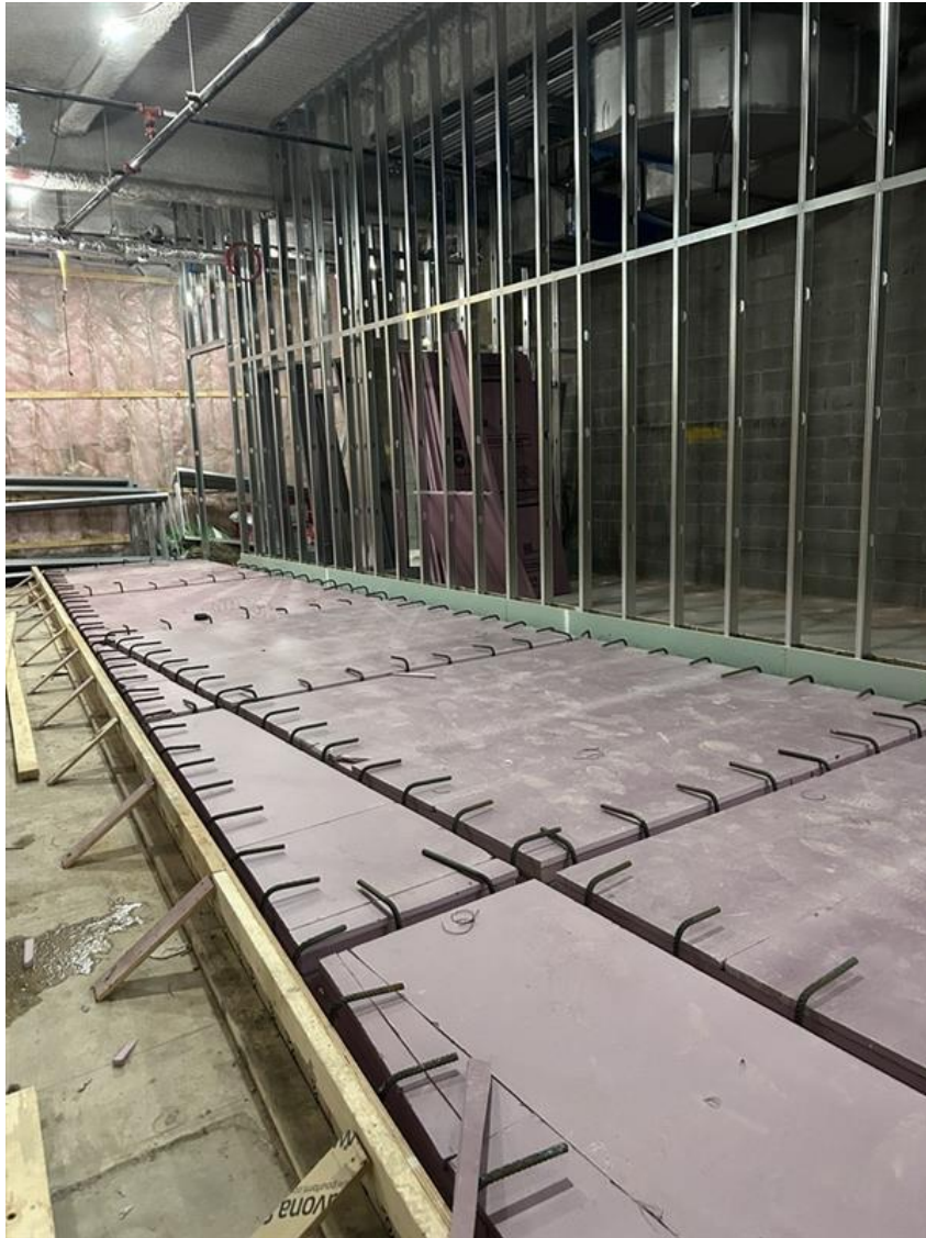
Foam and rebar installation in preparation for the Basement slab concrete pour.
