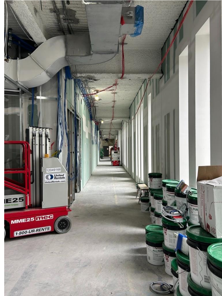
Ceiling conduit installation and painting are ongoing on the Podium floors.
