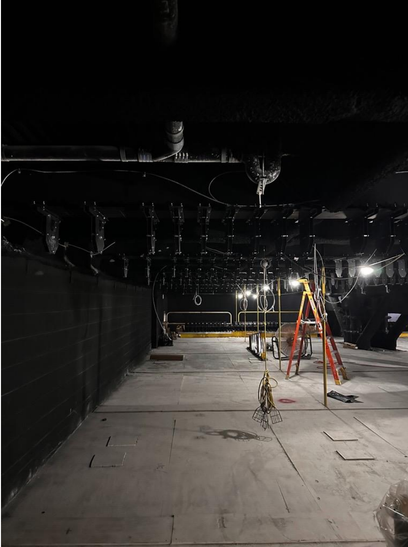
Schimmel Theatre Grid Iron – Loft Block installation.
