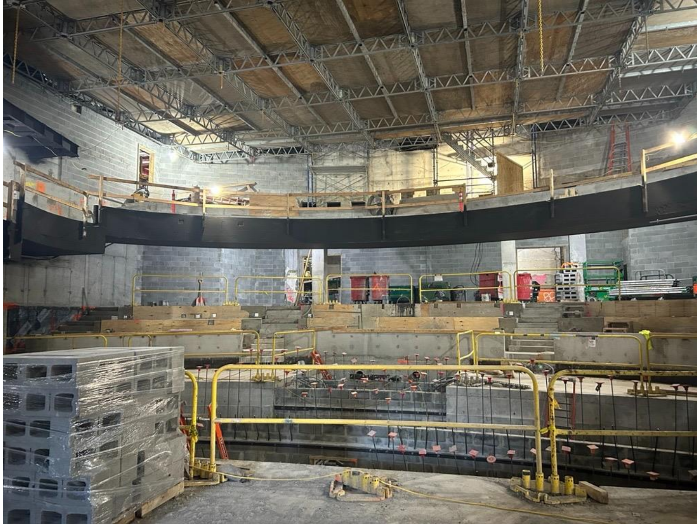
Progress in the Schimmel Theatre – lower seating well CMU installation.
