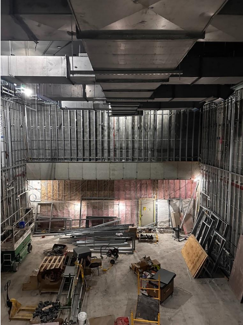
Small Venue framing and ductwork installation is ongoing.
