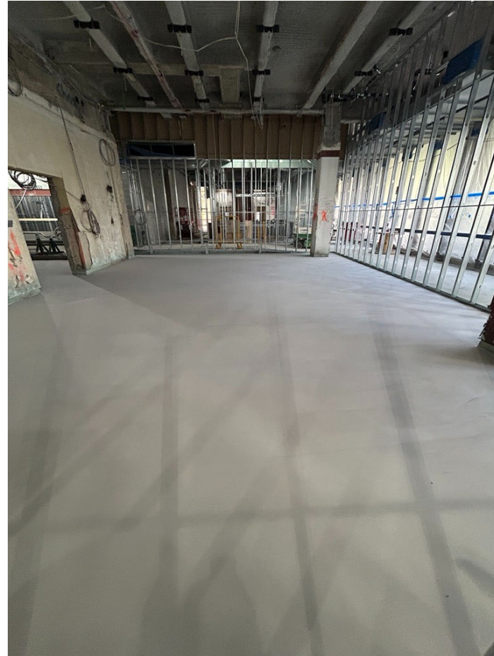
1 st Floor concrete topping slab installation.
