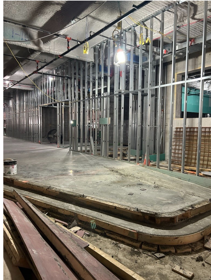
Framing on the ground floor continues along with topping slab pours outside of the Small Venue.
