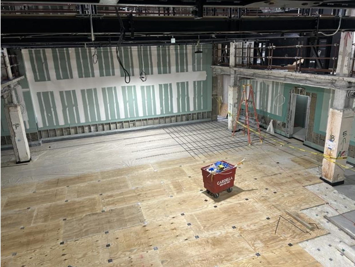
Specialty hardwood floors being installed in the Medium Venue.
