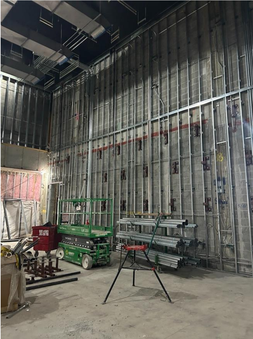
Small Venue rigging unistrut is being installed.
