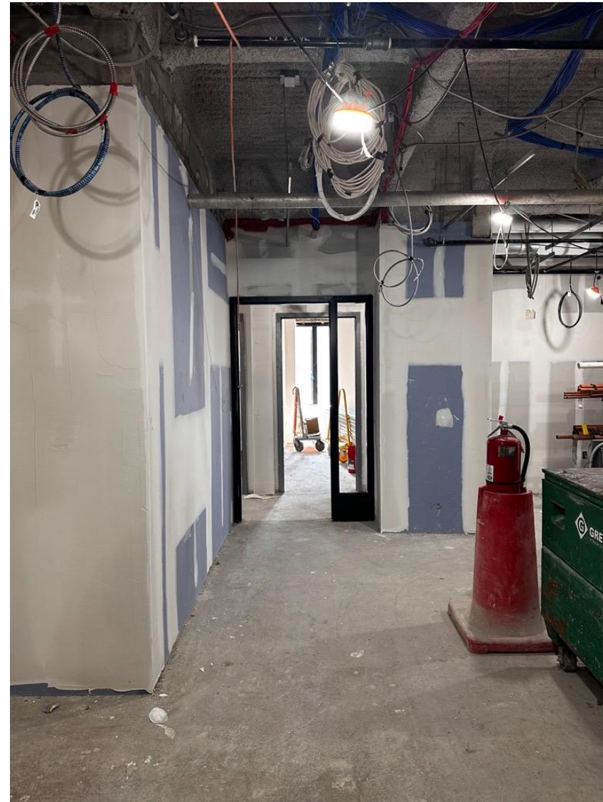
Maria's Tower 18 th Floor new walls and door frame installation.
