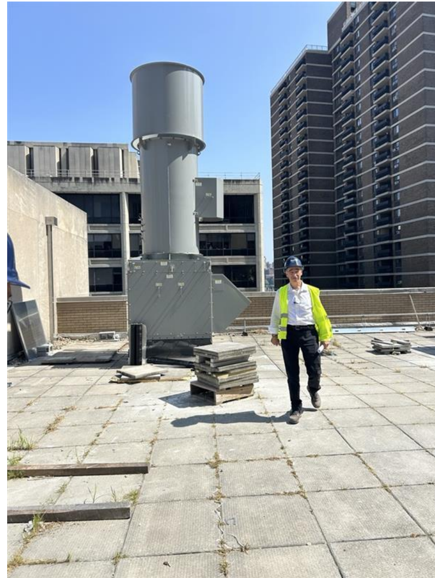
Exhaust for Spray-paint booth.
