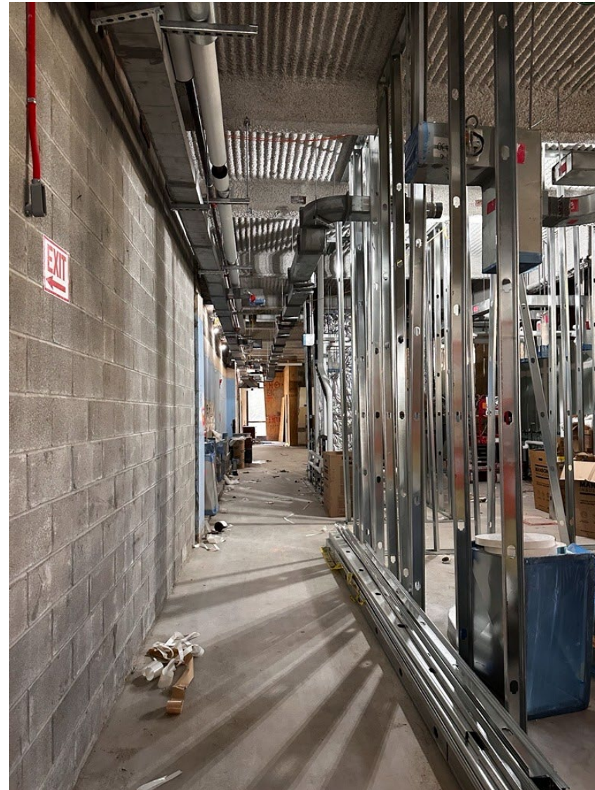
Framing and MEP installation throughout the Podium continue.
