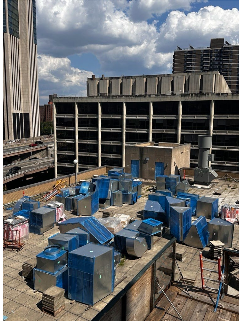
4 th Floor Roof - New ductwork that services new rooftop equipment.
