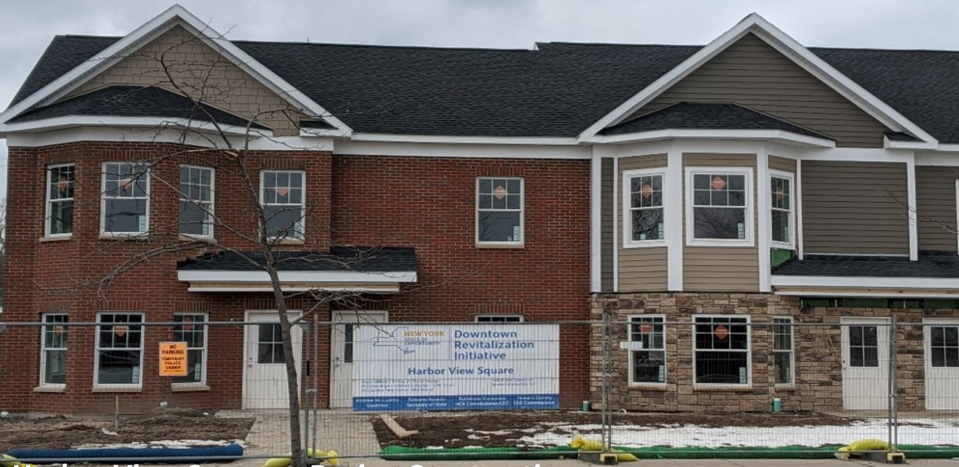
Harbor View Square—During Construction
