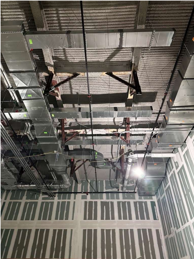
Installation of strong points in Large Dance Rehearsal is complete.
