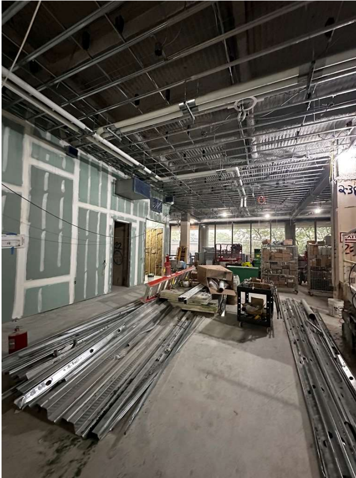
Installation of interior partitions, ceiling, and MEPs in continuing in the new Scene Shop.
