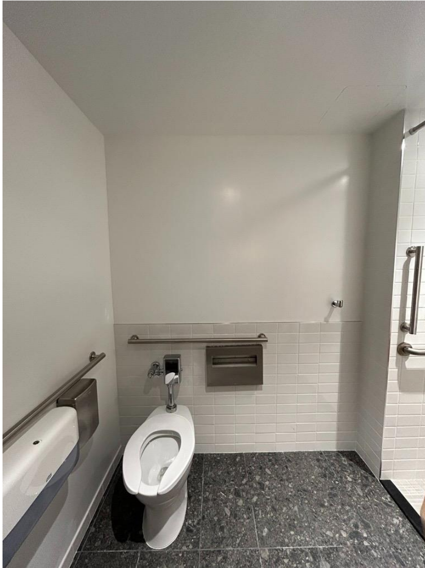
Maria's Tower Bathroom accessories have been installed for the mock-up bathroom.
