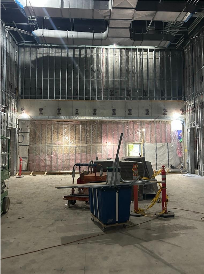
Small Venue overhead conduit installation is ongoing.
