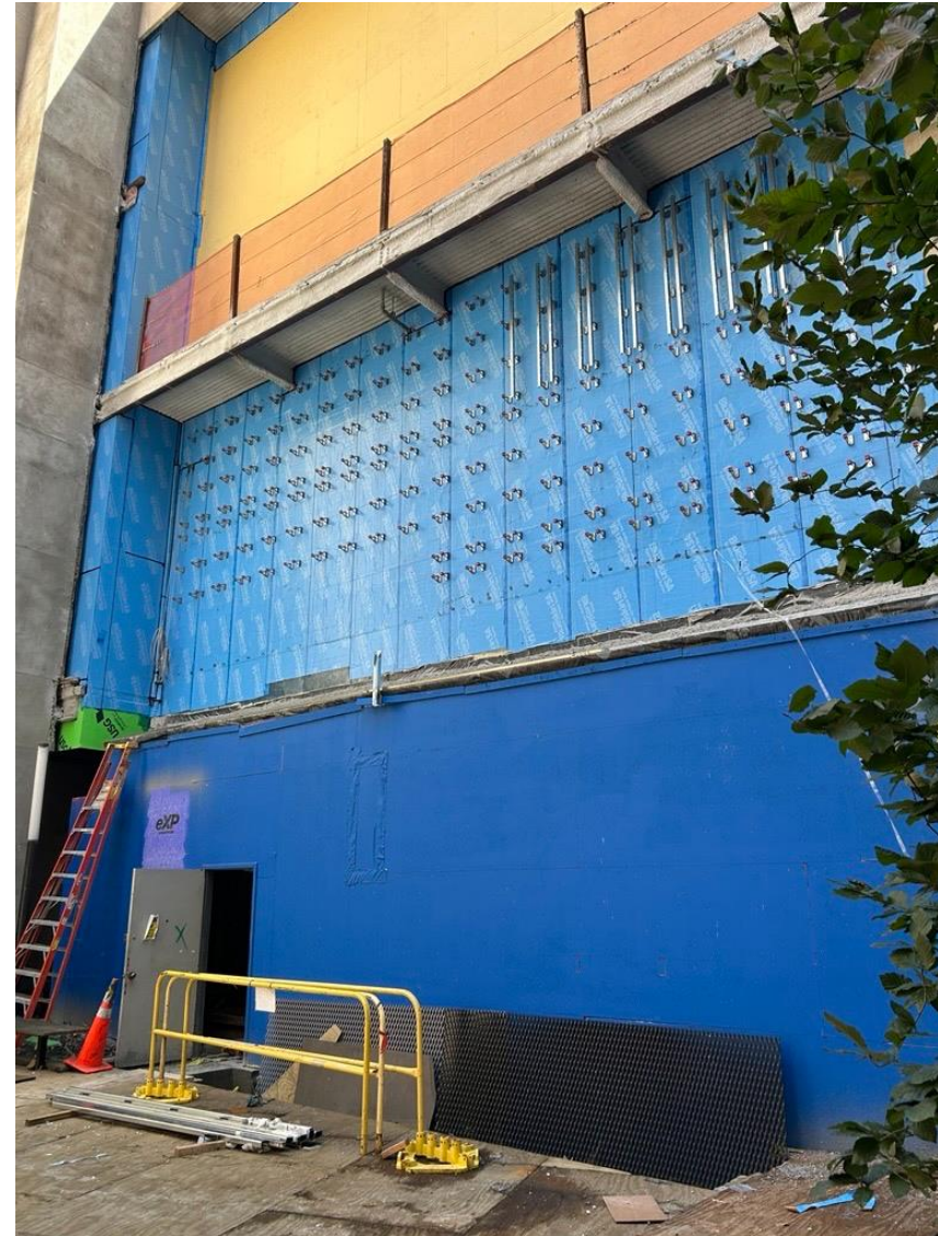
Courtyard East Elevation waterproofing installation is ongoing.
