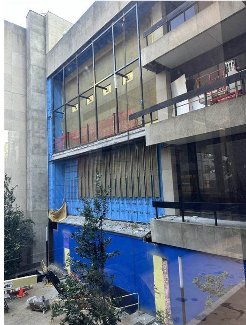
Ongoing installation of new exterior façade systems on Gold St and Courtyard.
