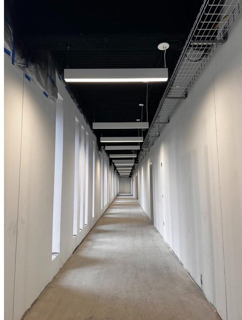
Podium light fixture and cable tray installation continues throughout corridors.
