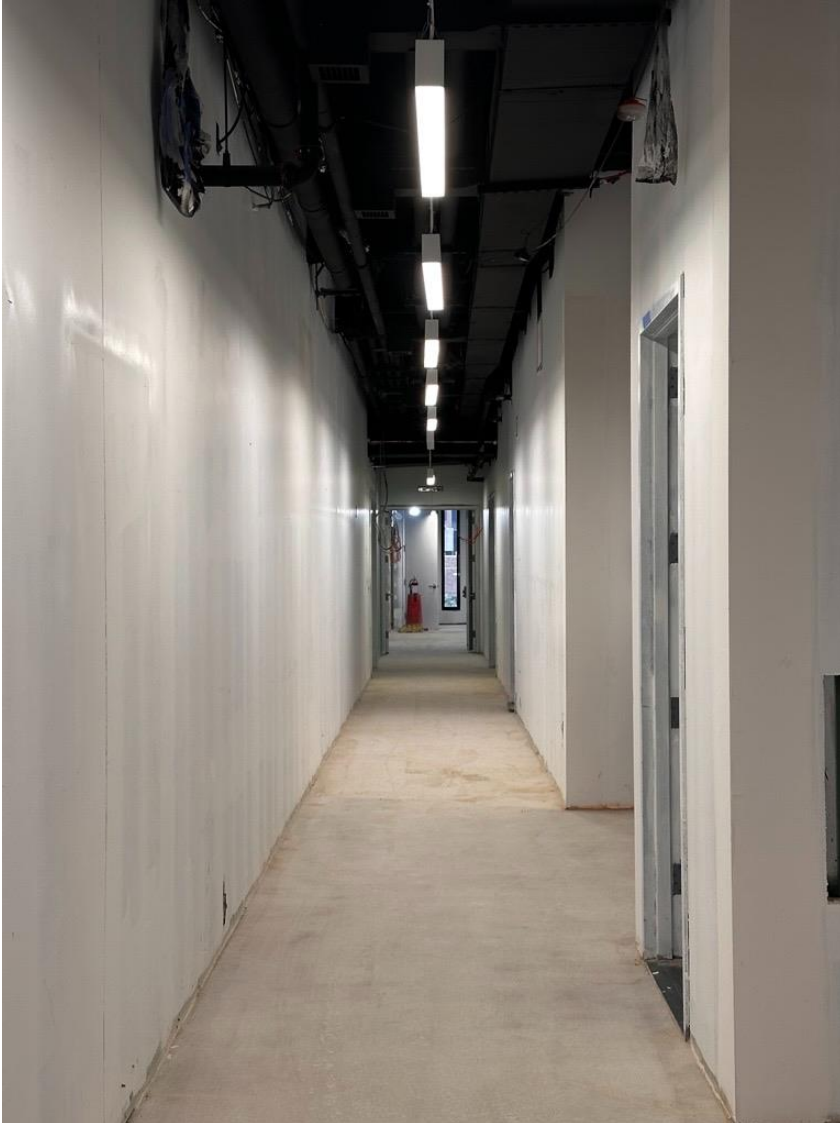
Podium light fixture and cable tray installation continues throughout corridors.
