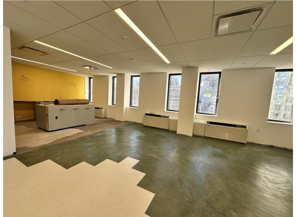
18 th Floor Residential Amenity Space Floor Installation Progress.
