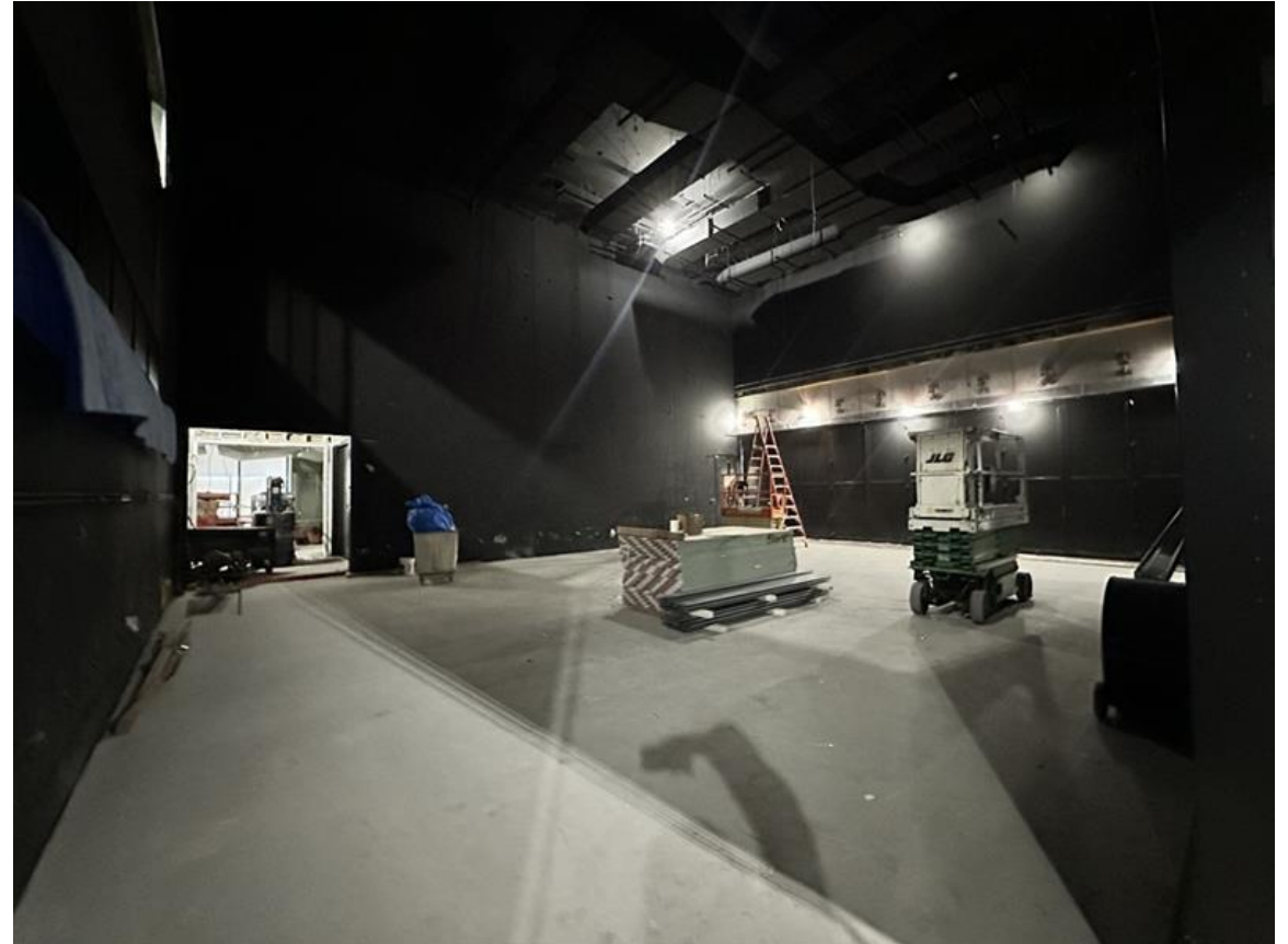
Garden Theater progress.
