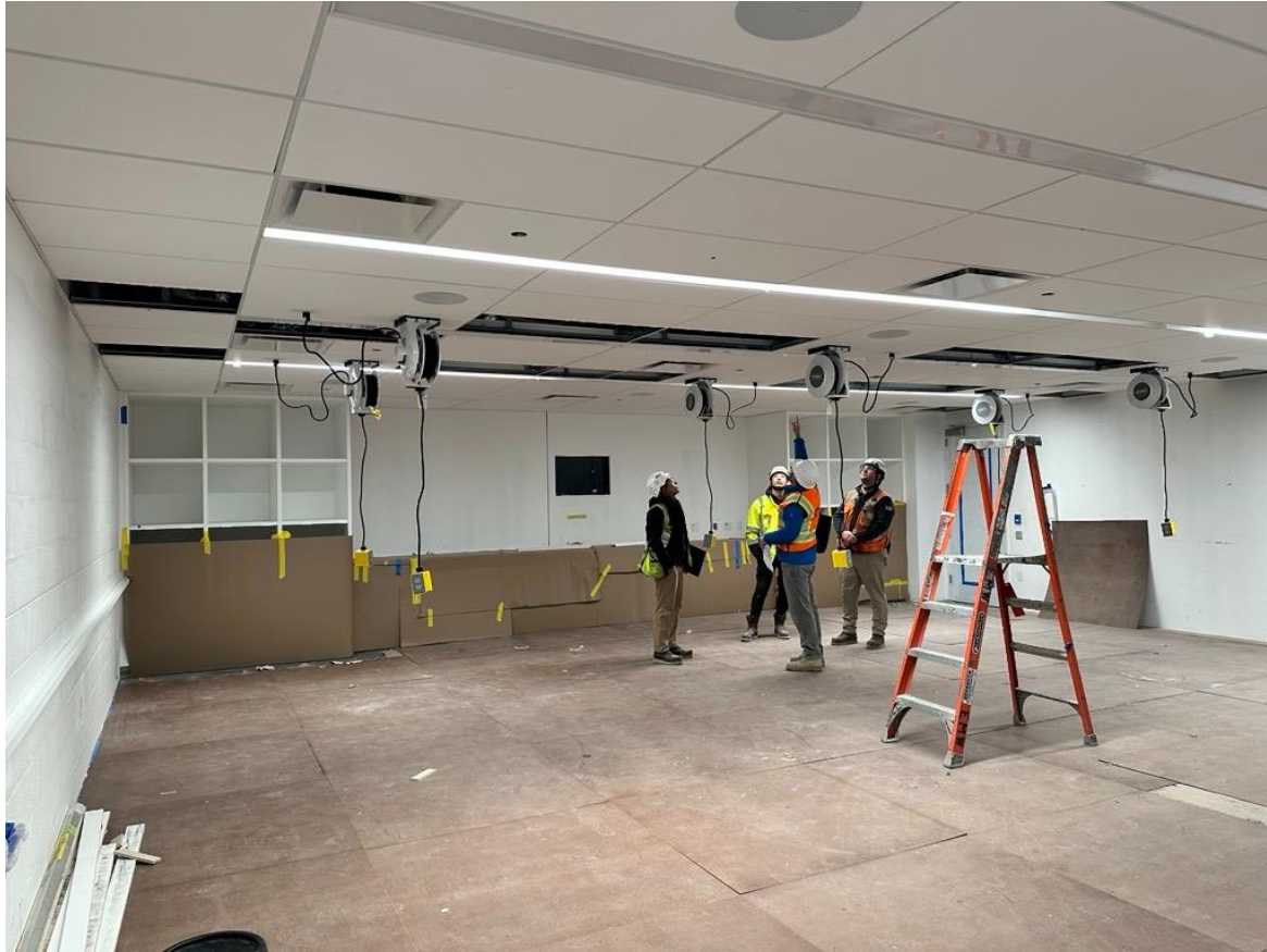
University Markerspace progress.
