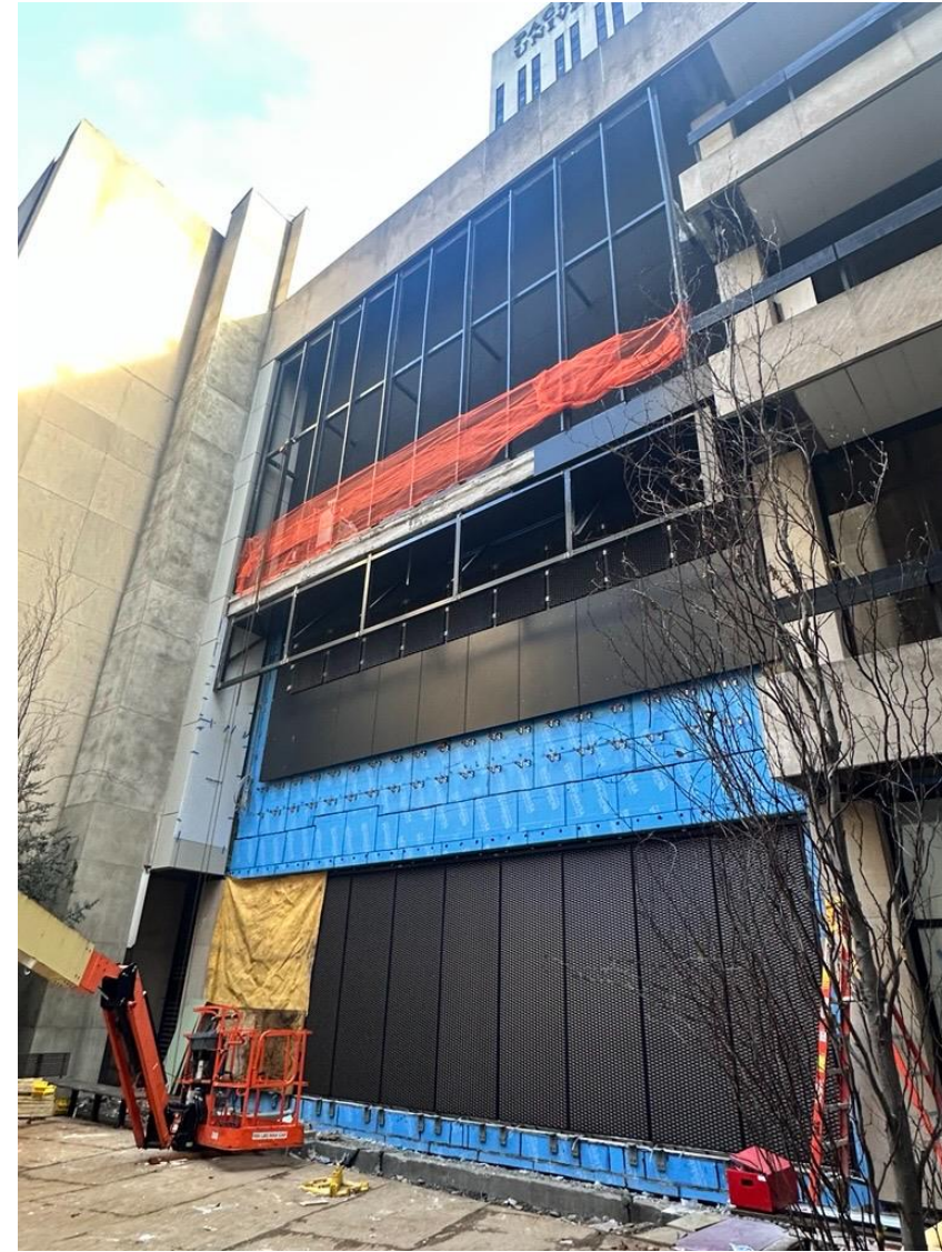
Courtyard façade progress.
