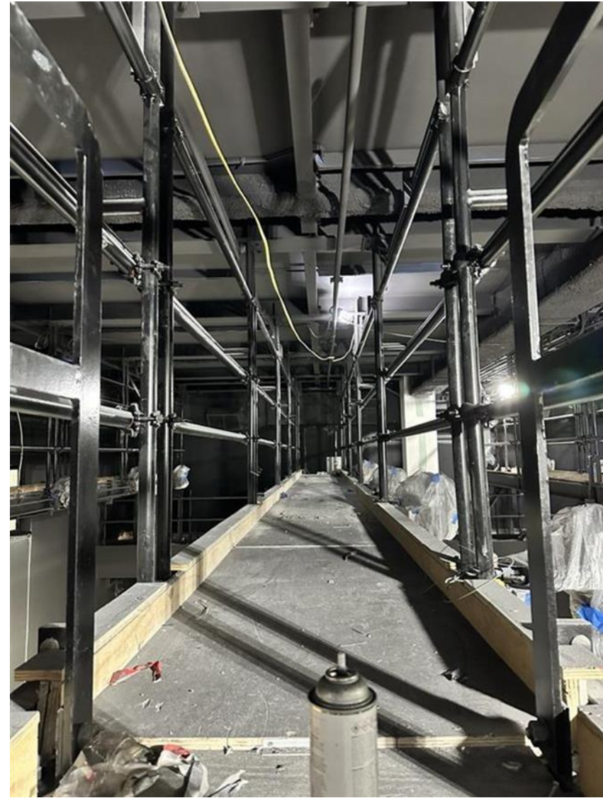
BlackBox Theater catwalk progress.
