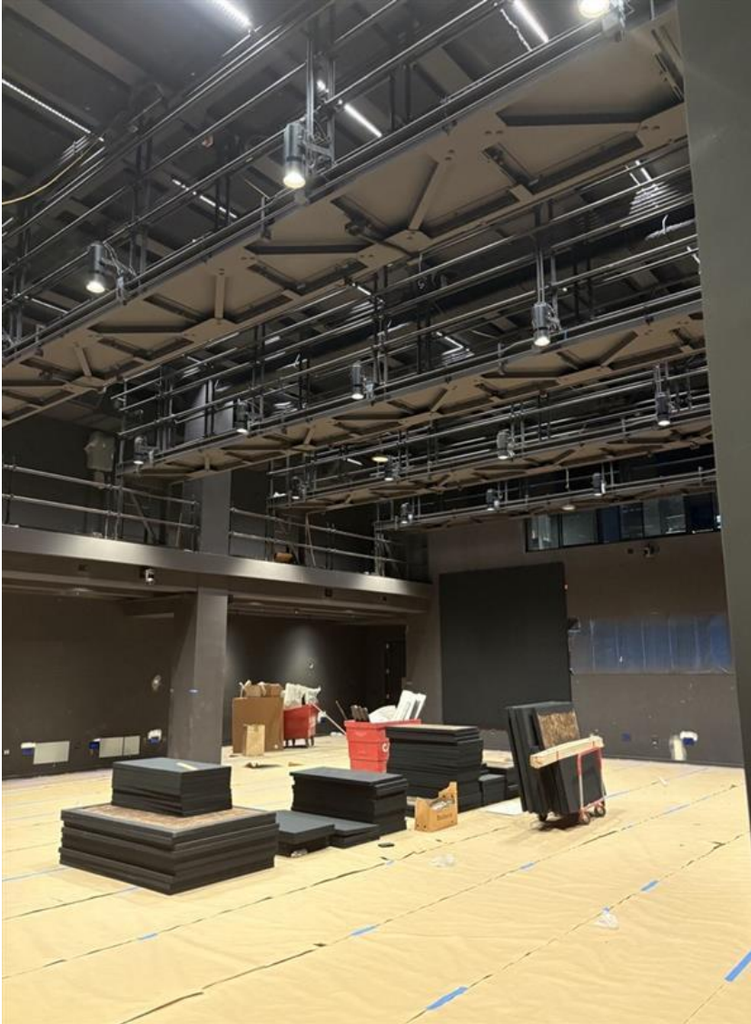
BlackBox Theater progress
