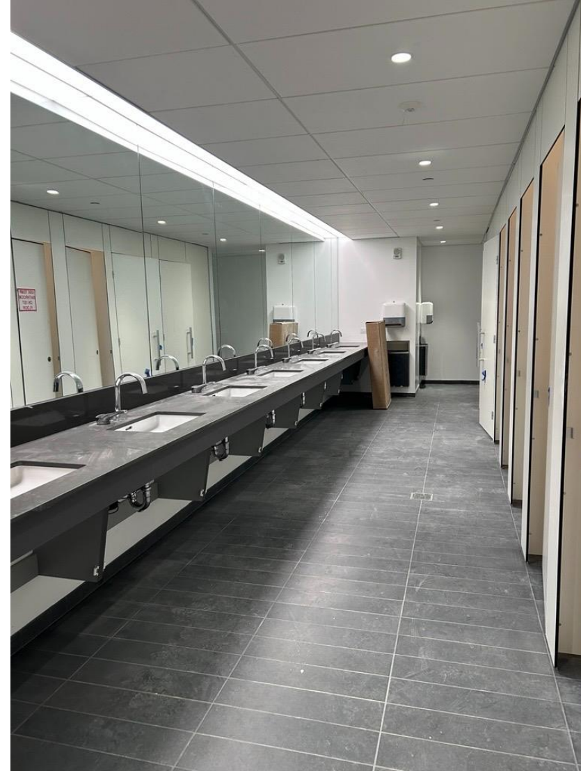
Restroom punchlist ongoing
