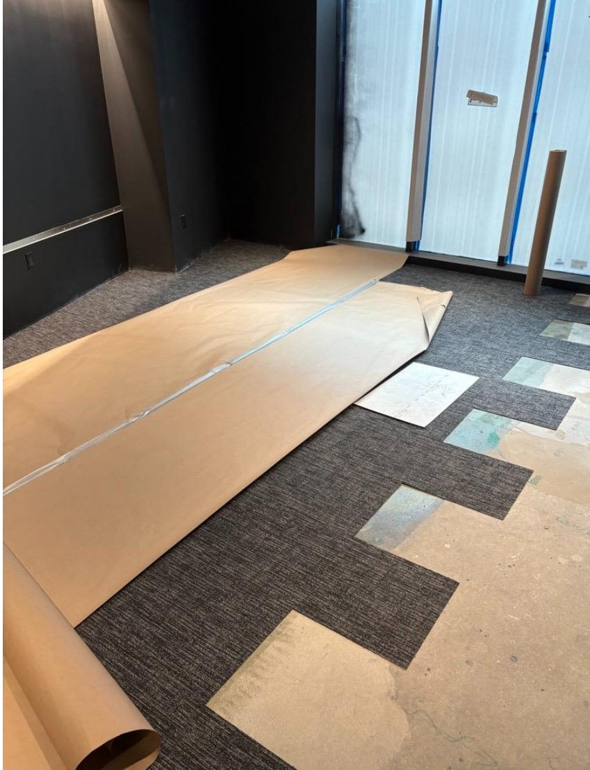
Carpet installation ongoing in 2 nd floor lobby corridor
