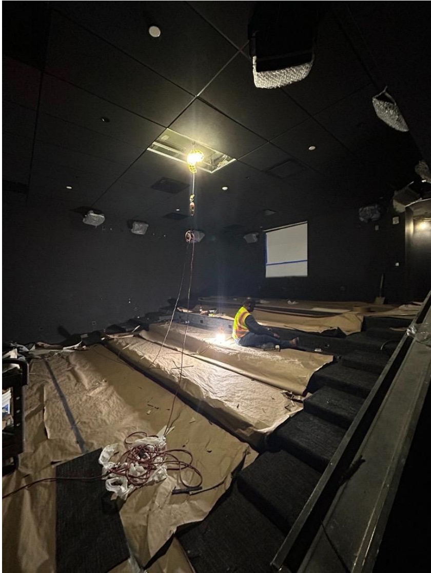
Screening Room progress
