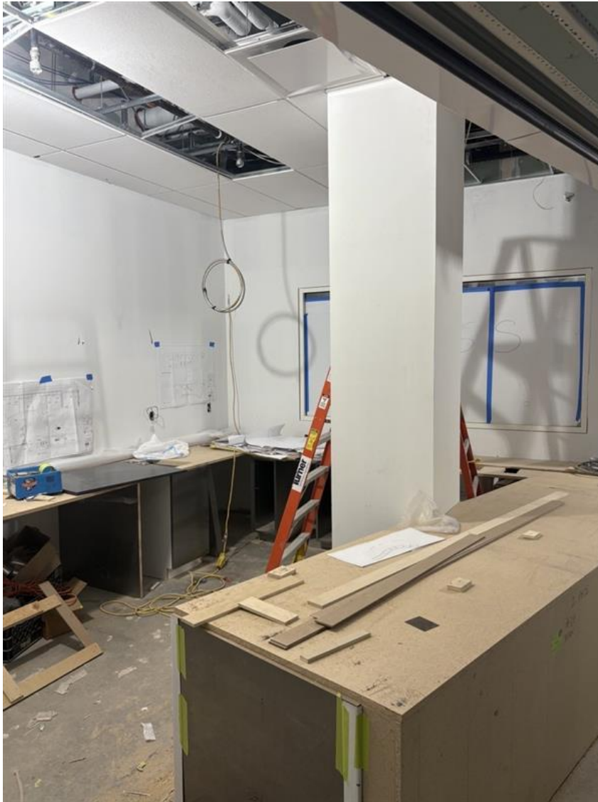
Café millwork installation ongoing
