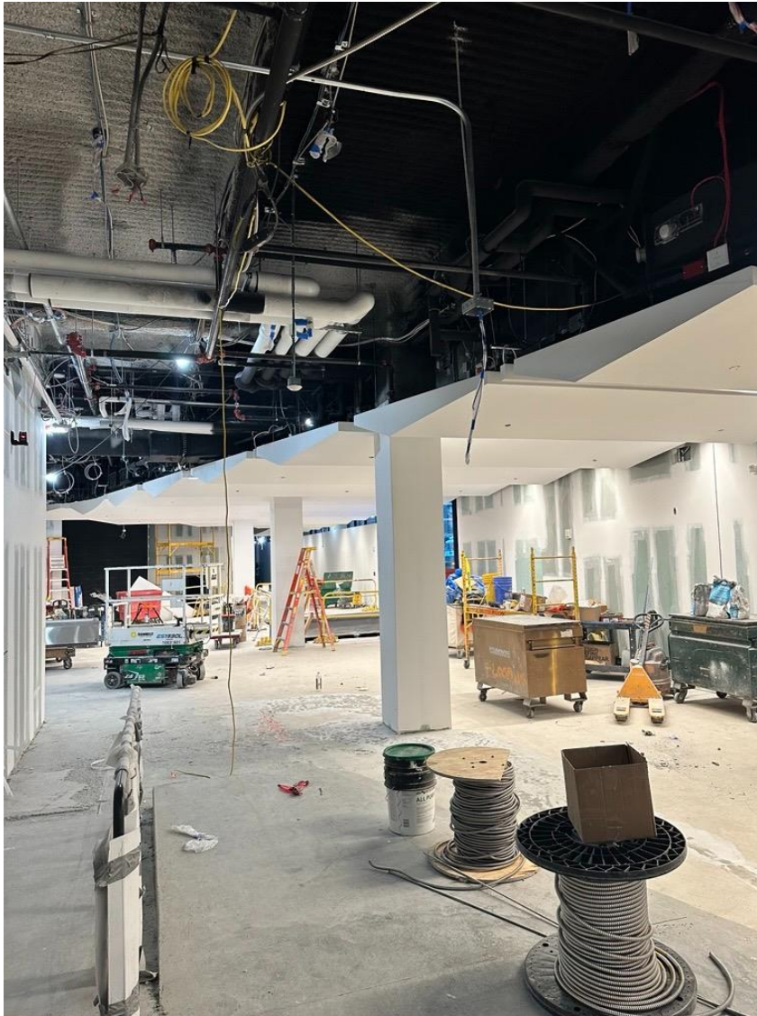
Garden Level Lobby progress.
