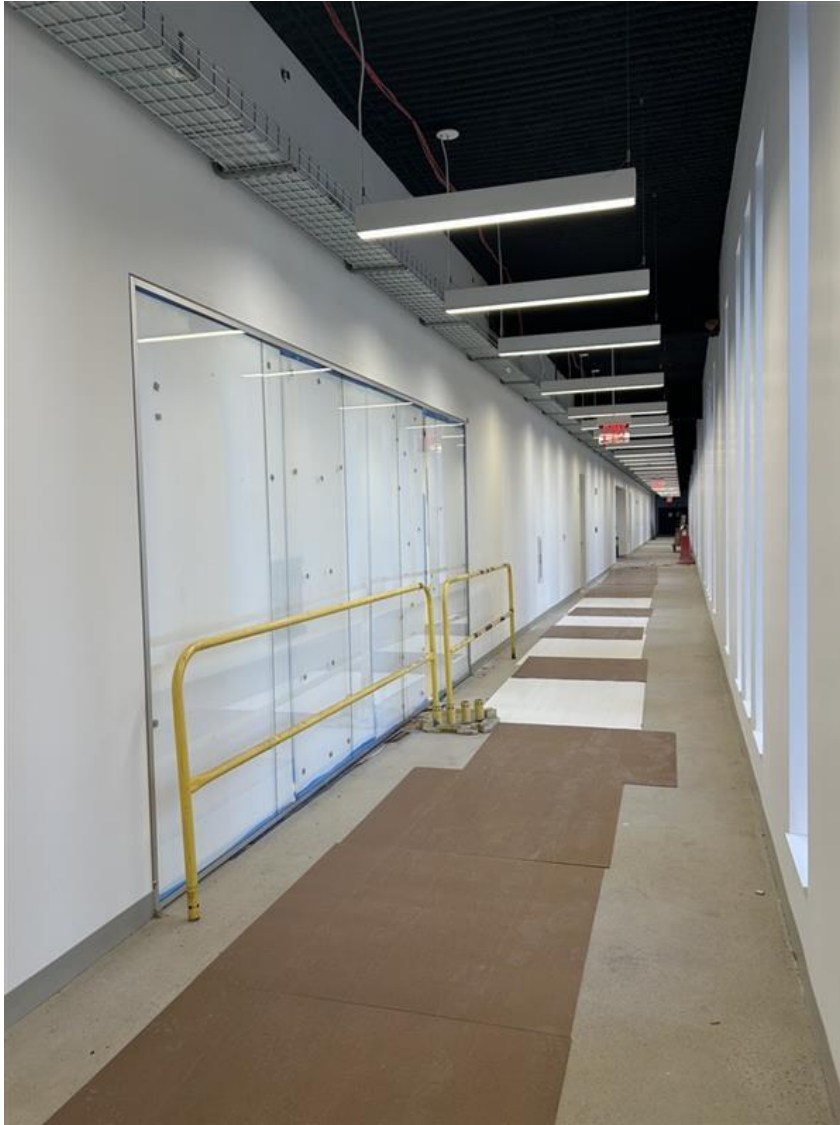
3 rd Floor Corridor Outside of Costume Shop.
