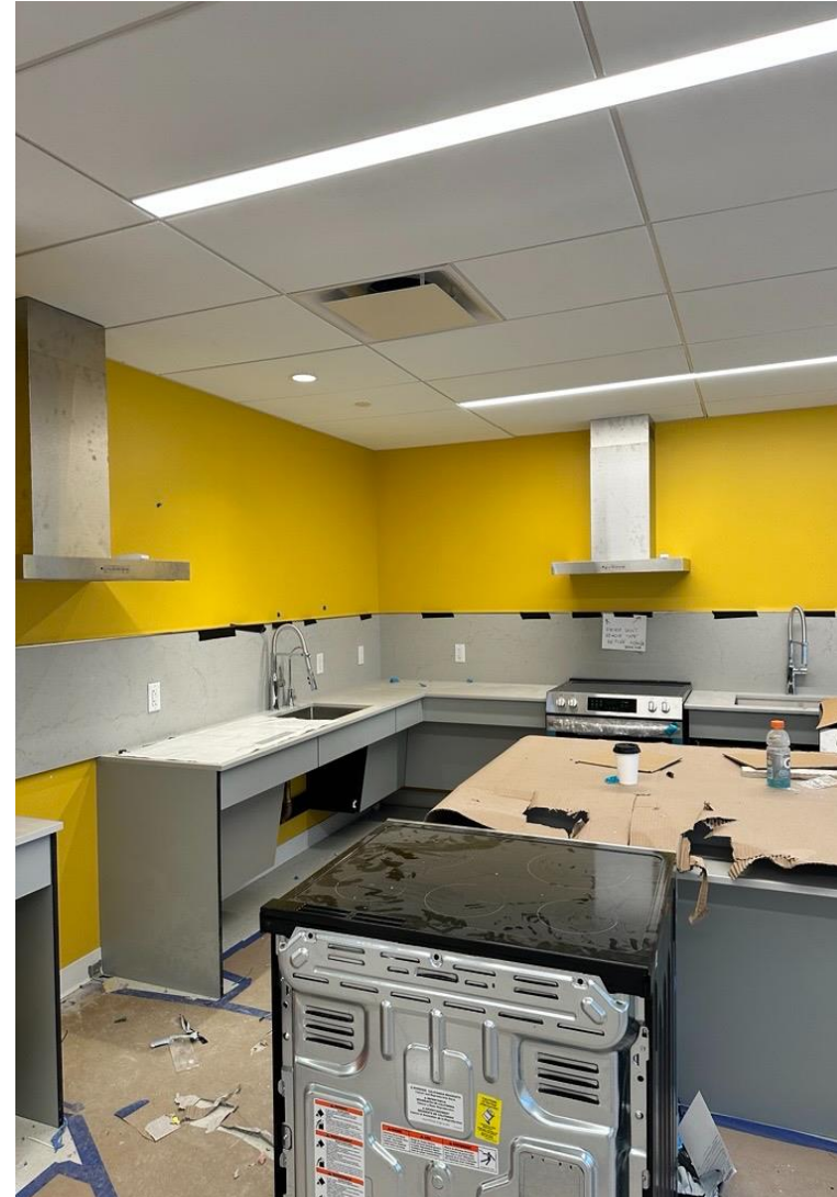
L18 Student Lounge – Kitchen Appliance Installation
