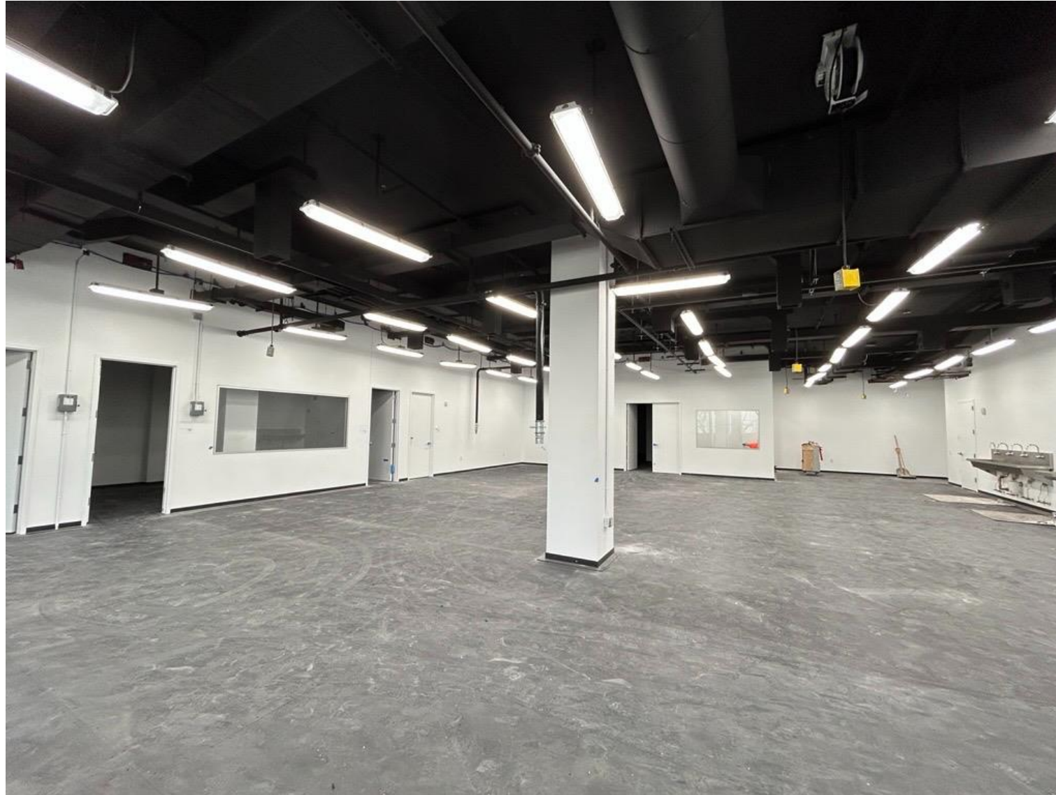
1 st Floor Scene Shop progress
