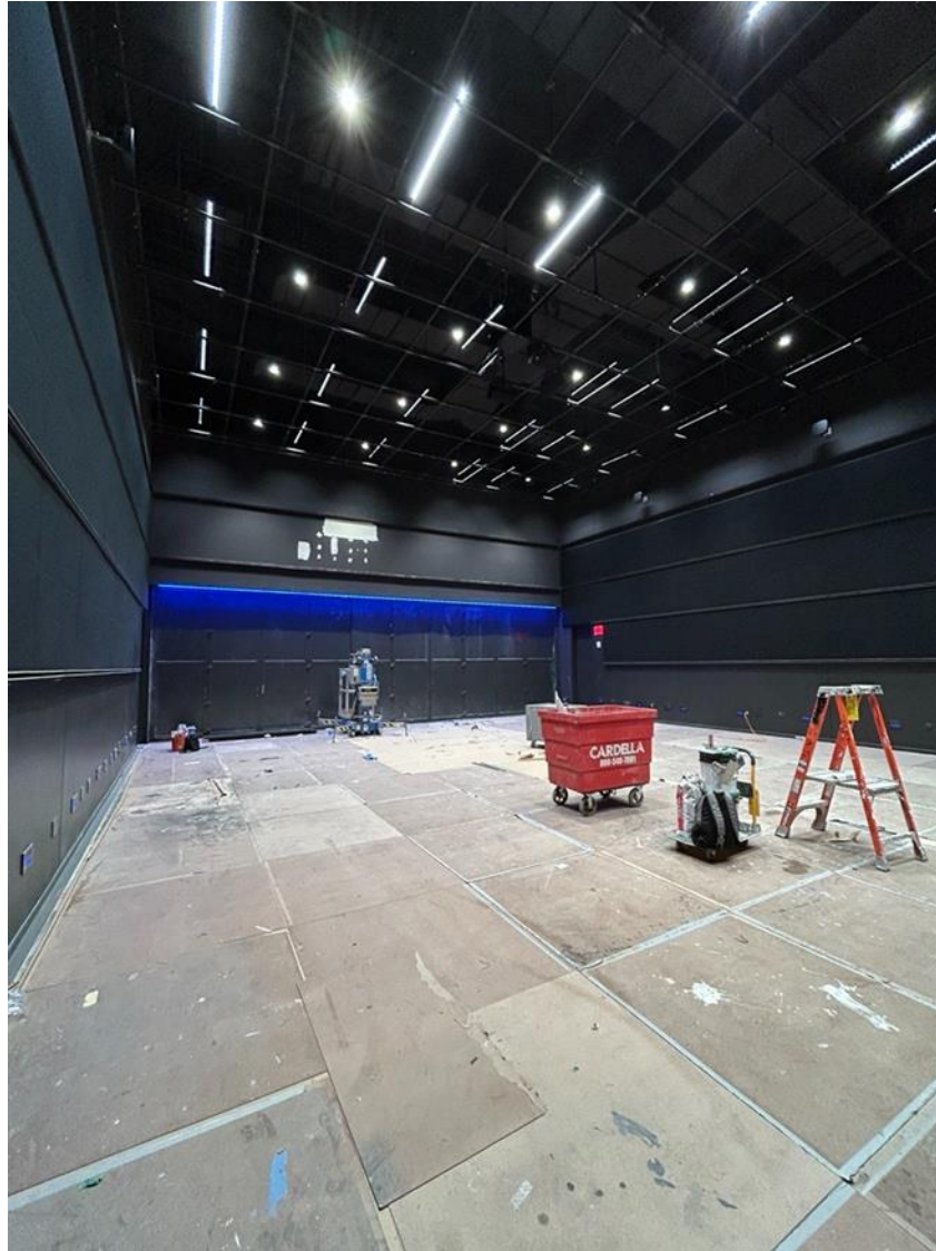
Small Venue commissioning is ongoing
