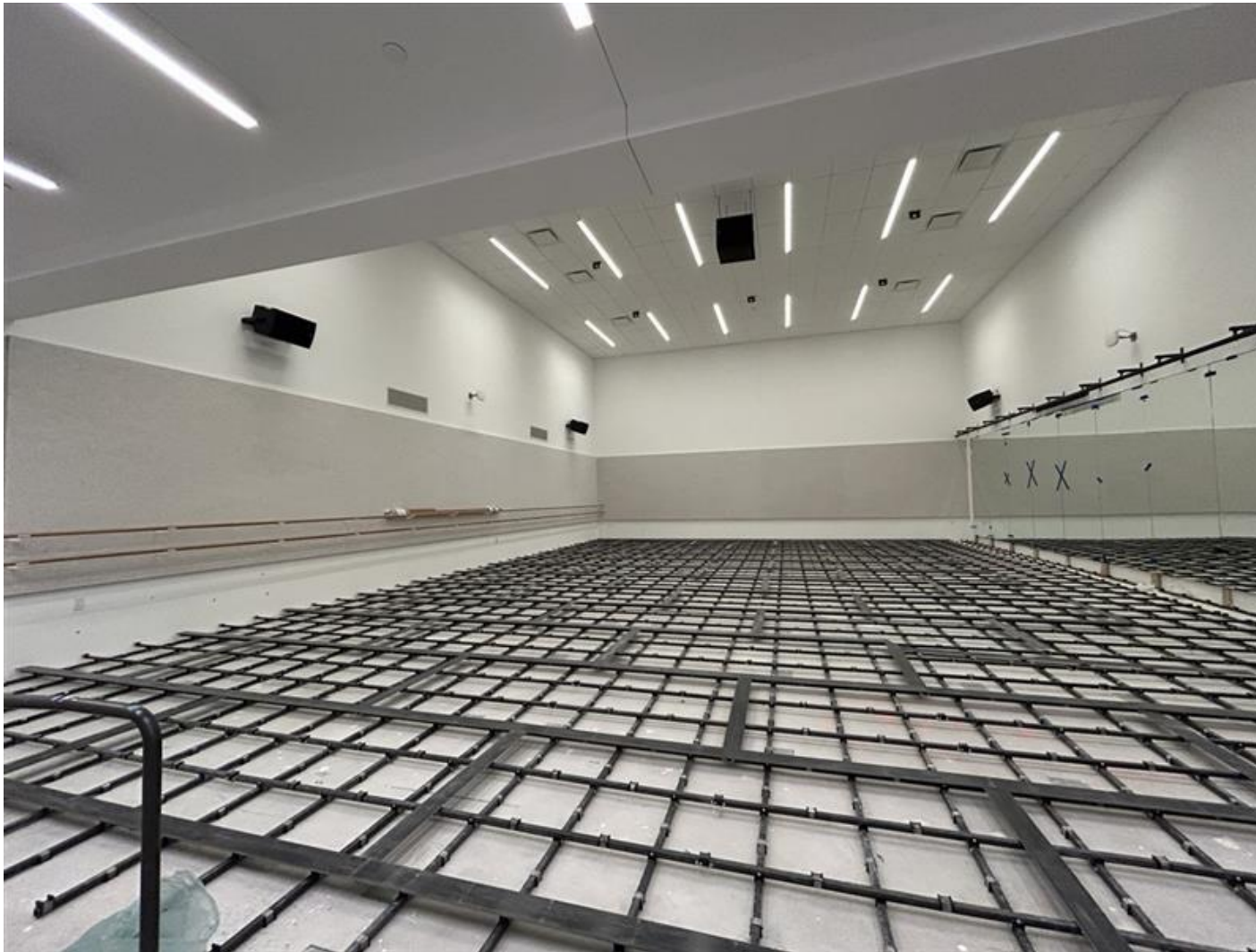
Large Dance Rehearsal FiberSprung flooring installation is ongoing
