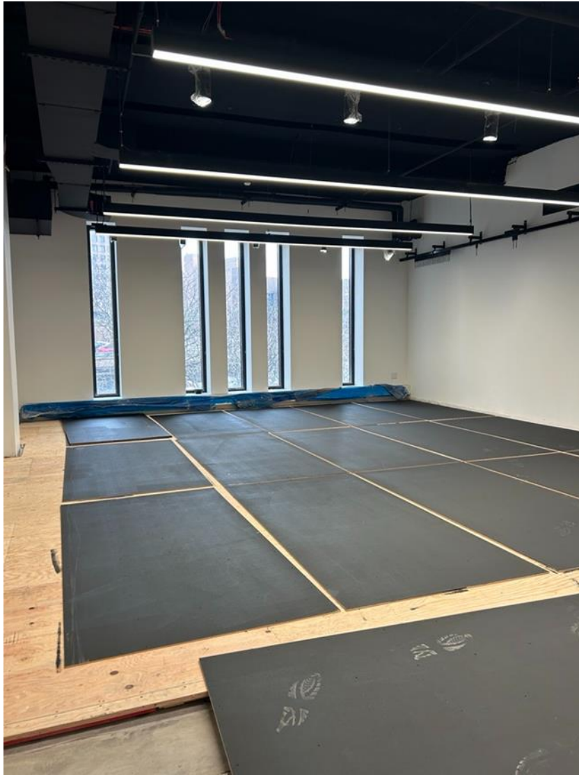
Level 2 Rehearsal Room Floor Installation
