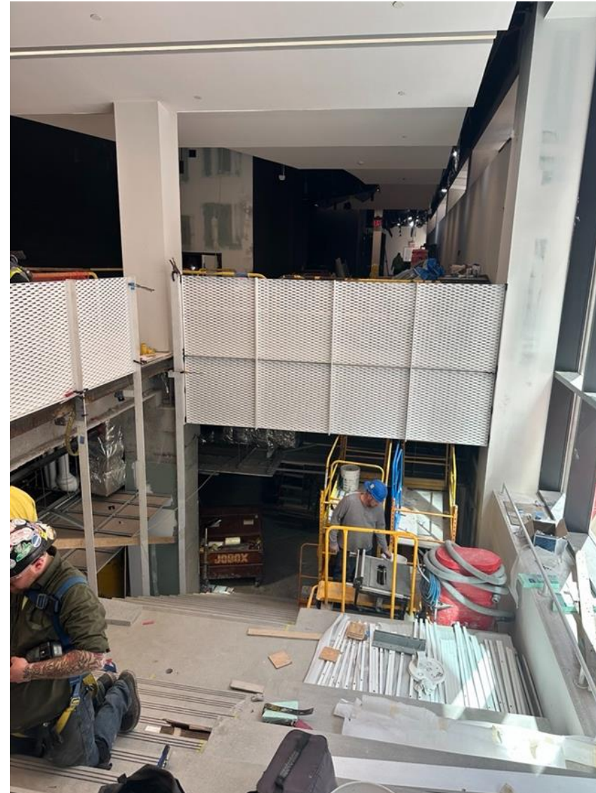
Spruce Street Stoop Ornamental Mesh Installation
