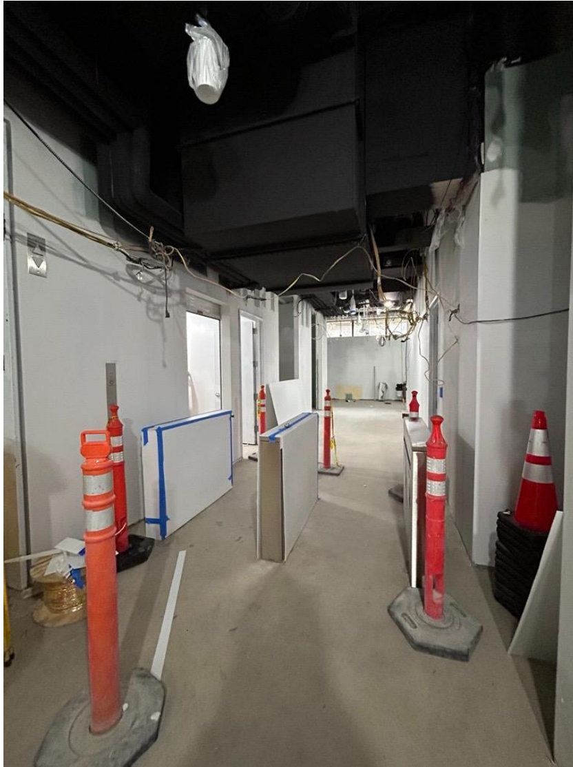
Residential Entry Turnstiles Installation
