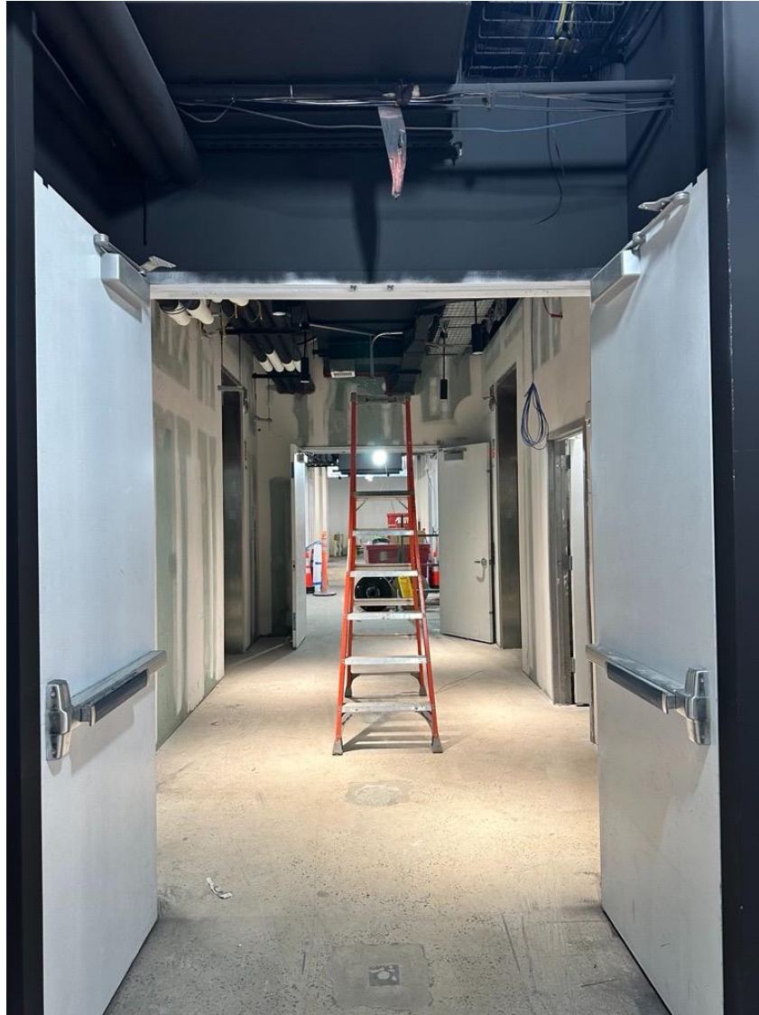
Garden Level Elevator Lobby Progress
