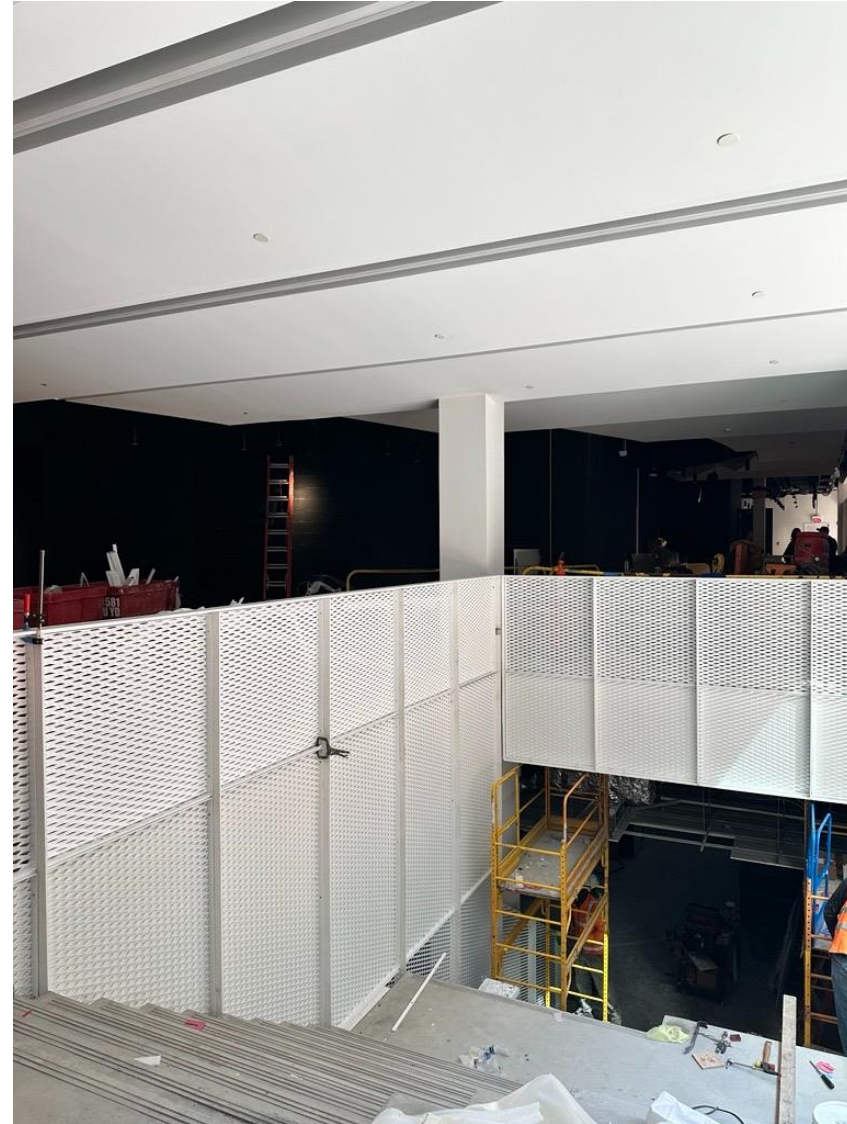
Spruce Street Stoop Ornamental Mesh Installation
