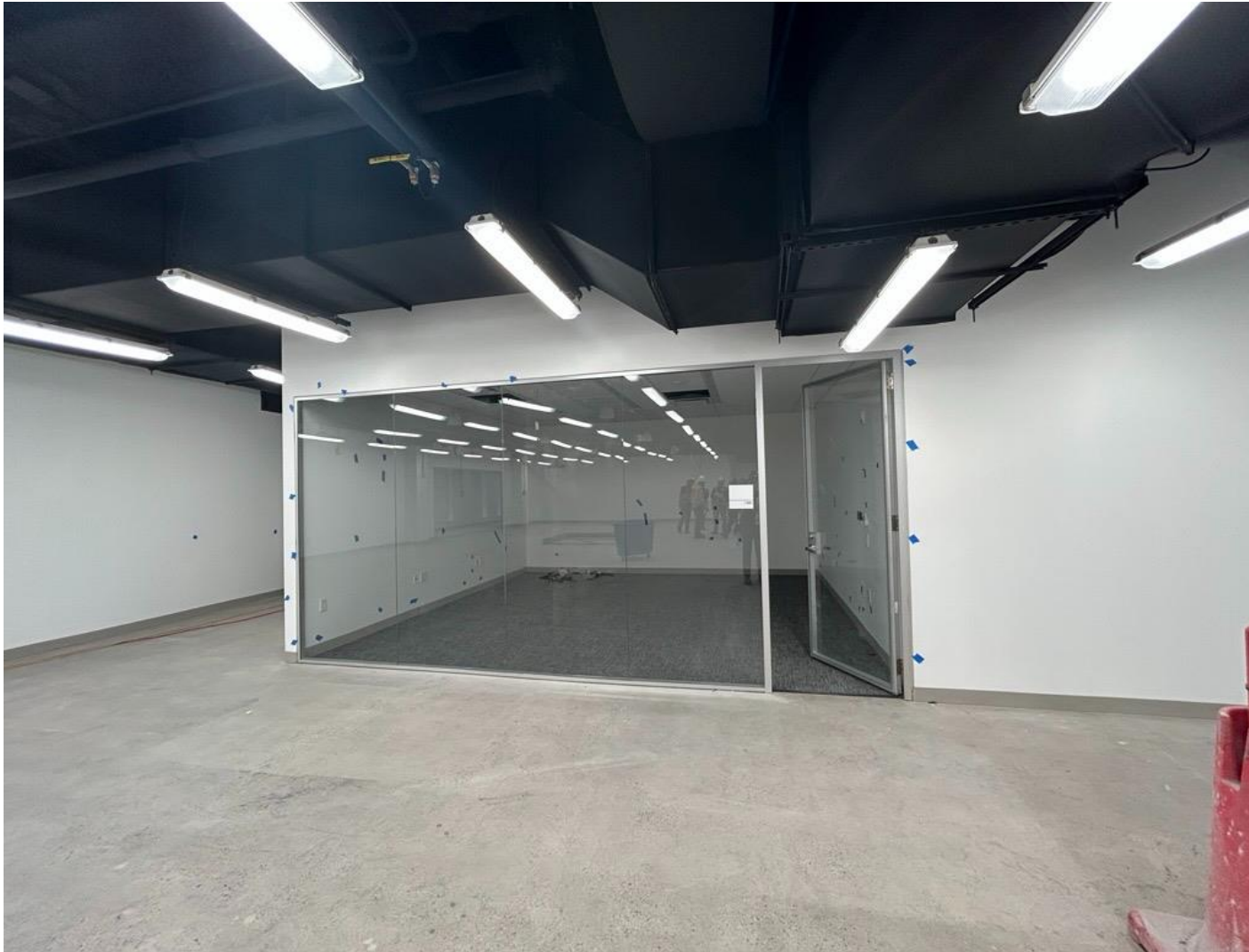
Level 3 Costume Shop Office Progress
