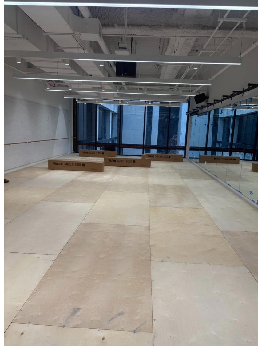
Small Dance Rehearsal FiberSprung flooring installation
