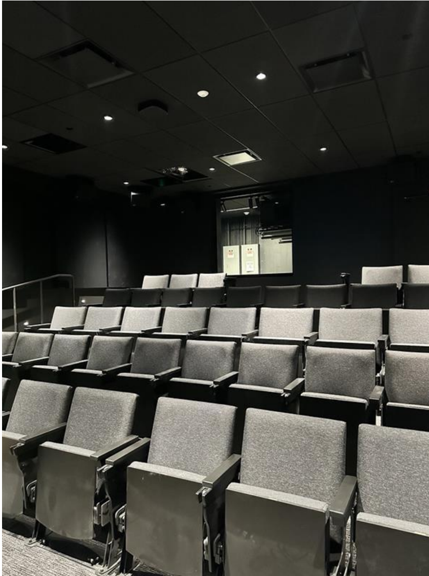
Screening Room progress.
