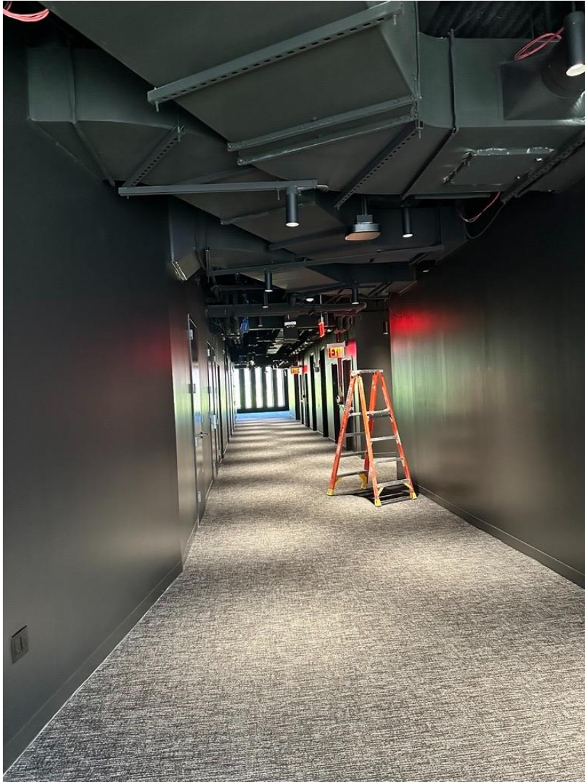
2 nd Floor Elevator Lobby progress.
