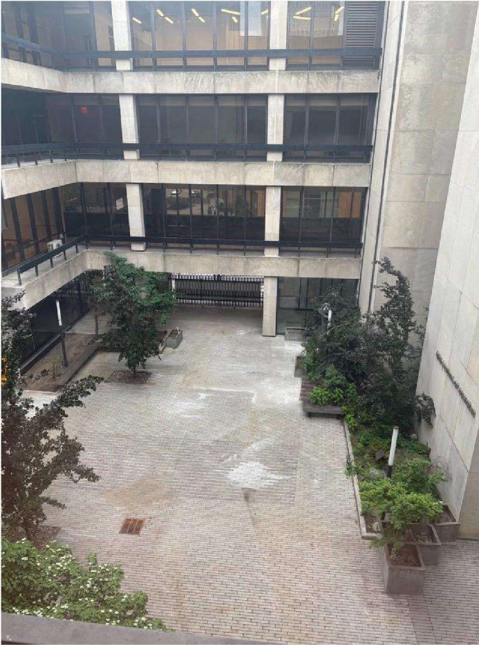
View to Courtyard from 2 nd Floor Offices
