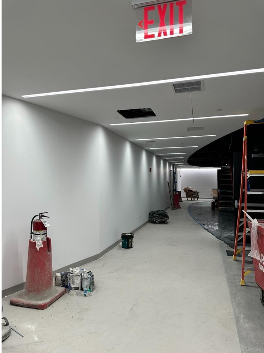
Schimmel Theater Pre-Function Lobby.
