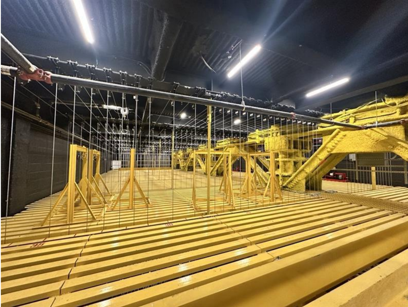
Schimmel Theater gridiron progress.
